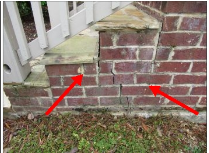
Brick movement at front steps
