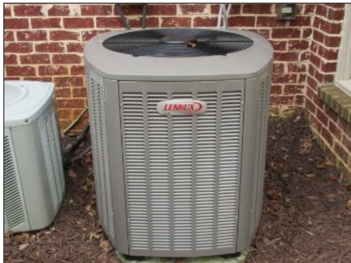
Second floor high efficiency AC unit
