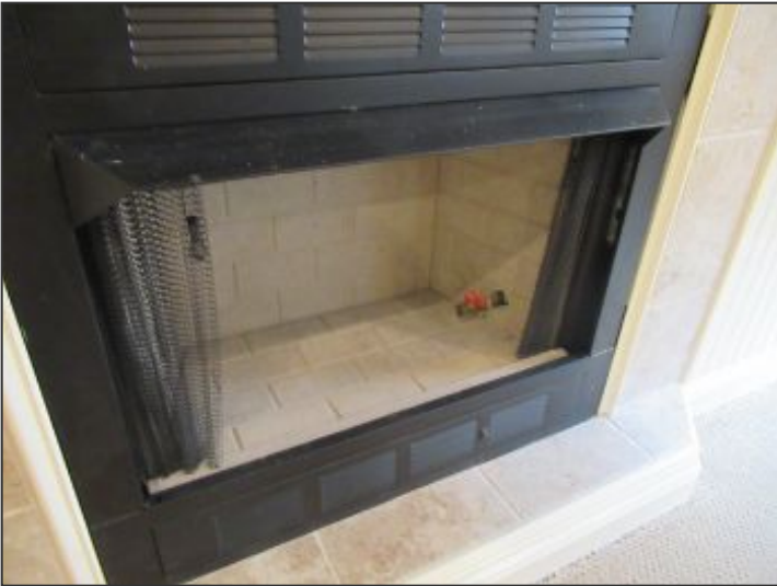
Basement fireplace logs have been removed
