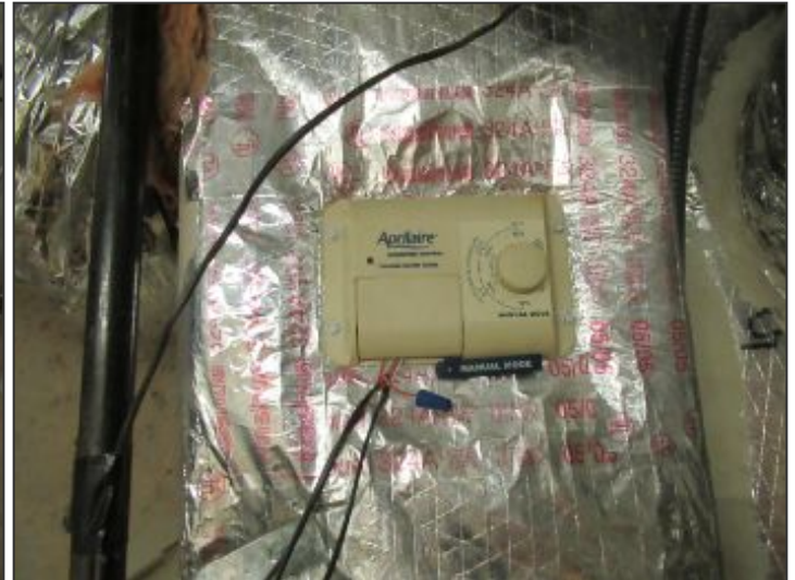
Humidifier not inspected
