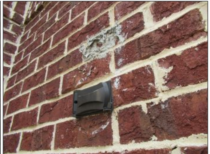
Basement doorway light removed
