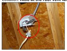
All electrical splices and terminations should be inside of an approved junction box
