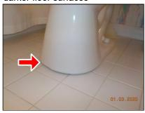
Toilet should be sealed between the base and floor
