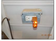
GFCI device failed to trip when tested
