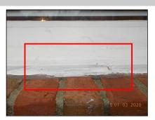
Wood rot and deterioration are present.
