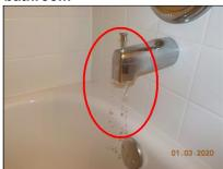
Shower diverter does not seal completely when engaged.
