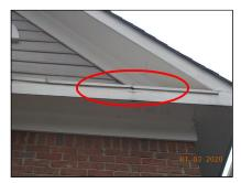
Wood rot and deterioration of the fascia board noted.
