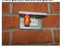
GFCI device failed to trip when tested
