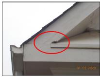
Wood rot and deterioration of the fascia board noted.
