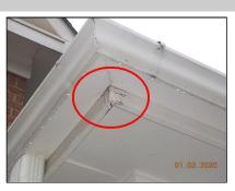
Wood rot and deterioration of the fascia board noted.
