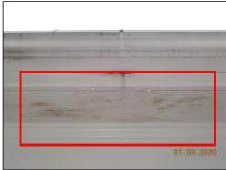
Wood rot and deterioration noted in the soffit.
