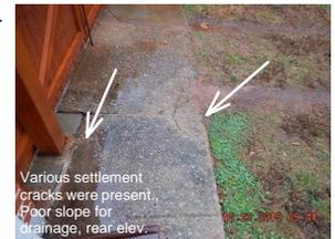
3. Steps/Stoops: Concrete - Uneven step riser height variation, slight trip hazard., Openings in front elevation guard rails >4", the current maximum spacing standard.
