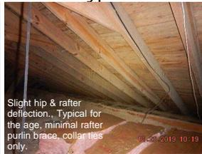
4.  Sheathing: Dimensional wood - Minor decking damage.
