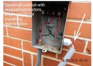
Detached conduit with exposed conductors., Slight conductor sheathing deterioration.
