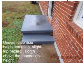
4. Porch: Concrete - Front & rear porches were installed above the foundation height. {typical} Moisture intrusion/termite concern., Openings in guard rails >4", the current maximum spacing standard.
