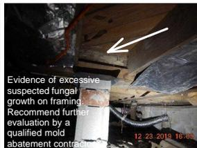
8.  Insulation: Not installed - Non-faced fiberglass insulation recommended after mold abatement.
