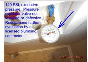
17. Water Lines: Thermal expansion device not located., Recommend further evaluation by a licensed plumbing contractor.
