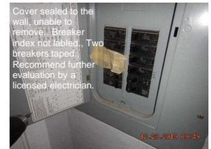
15. Interior-Hallway Electric Panel Breakers: Copper and Aluminum - 2 breakers were taped off., Index not labeled., Recommend further evaluation by a licensed electrician.
