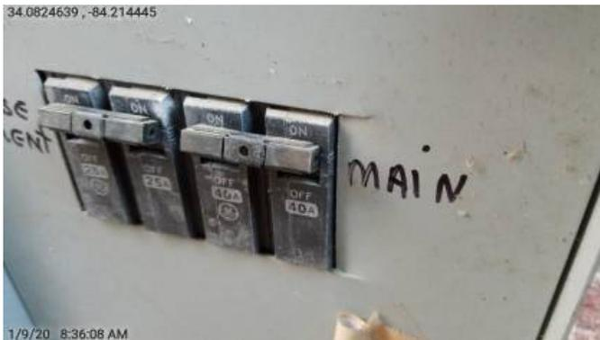
7.36 Capacity / Approx. Age:     3.5 Tons, Max Fuse: 40 amps, Brand, Trane brand, Manufacture Date- 2011.
