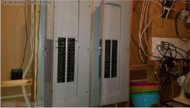
6.4 Main Circuit Rating And Service Disconnect:     Main Circuit Sizing: 300 amps. (2 x 150 amps).
