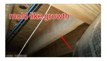
4.9 Beams/Underfloor:  $\square$ The floor joist system is constructed of: Solid wood floor joists.
