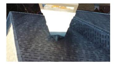
3.21 Chimney Cap:  $\overline{\mathbf{A}}$  The chimney cap is heavily rusted. This may indicate standing water (improper slope) and normal aging of the metal cap. This condition is conducive to water leaking into the chimney. Recommend treating the metal cap with an anti corrosive paint to halt the rusting process and ensure there is a proper slope on the cap for correct water management.
