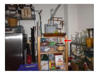
**Repair, Safety Issue:** The water temperature at the faucets/showers was too high (120 Degrees is normal). This condition can cause scalding and is an inefficient use of energy. Recommend adjusting the thermostat on the water heater to the correct settings for proper safety.
