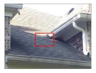
**Repair**: Split, loose or damaged ridge caps as noted at the left center require repair or replacement to prevent leakage.
