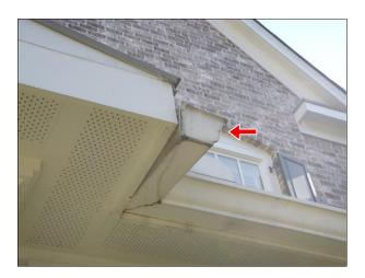
**Repair:** Leaks in the downspouts and gutters should be repaired by re-sealing the joints to prevent damage to the cornice. Have all connections inspected and repaired as necessary. The gutters and downspouts should also be checked for blockages and proper flow.
