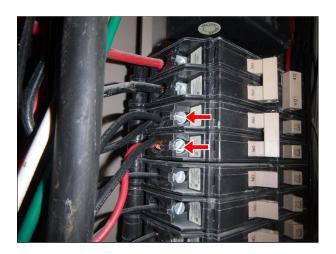
**Improve:** Missing screws as noted at the front panel cover of the main electrical panel should be replaced for proper securing of the cover. All screws attaching the panel cover should be blunt headed to prevent possible damage to the wiring.
