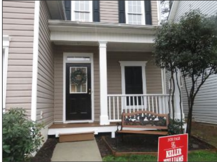
Wood porch at front entry
