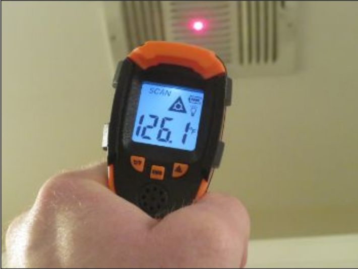
Gas furnace heating normally - 126 degrees
