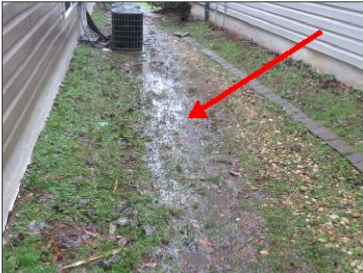
Standing water at left side yard
