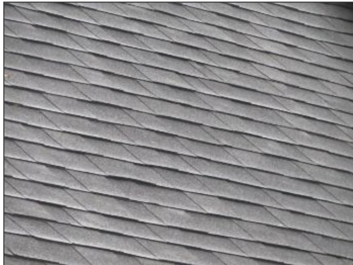
Architectural roof shingles present
