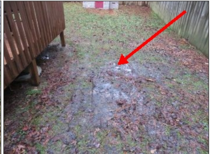
Standing water and excessively muddy conditions at rear right yard
