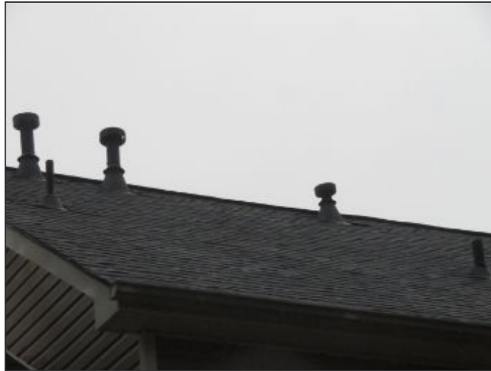
Rear roof surfaces look good
