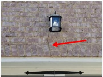
Minor brick crack at center of overhead garage door
