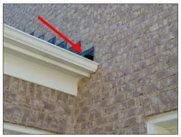
Good kickout flashing at roof intersections
