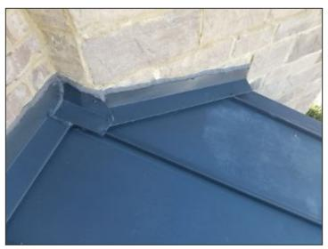
Front porch roof well sealed at wall connection
