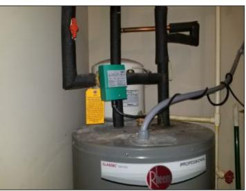
Recirculating pump present at water heater
