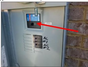
Main electrical disconnect at exterior meter
