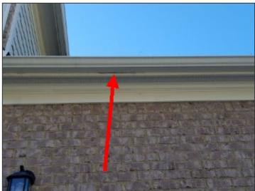
Damaged fascia at left side single car garage roof
