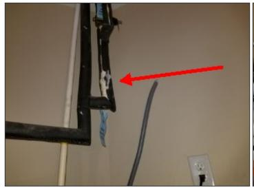
Main water cut-off handle located above water heater
