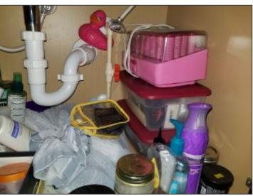
Rear wall hose bib cut-off handle located below shared bathroom sink
