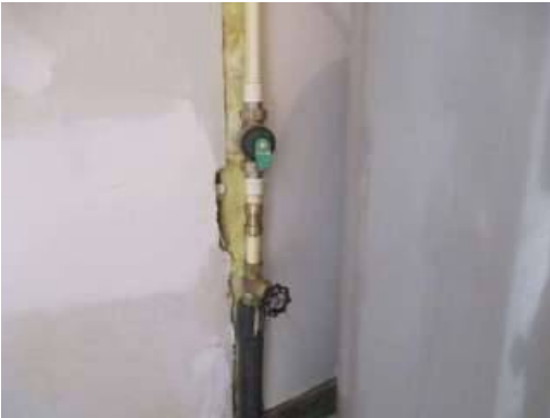
Photo 51-1 Garage utility room
