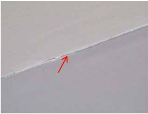
Photo 43-3 Top level front bedroom at ceiling
