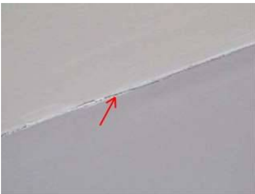
Photo 43-3 Top level front bedroom at ceiling
