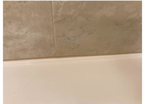
Master Bathroom 3rd Floor
