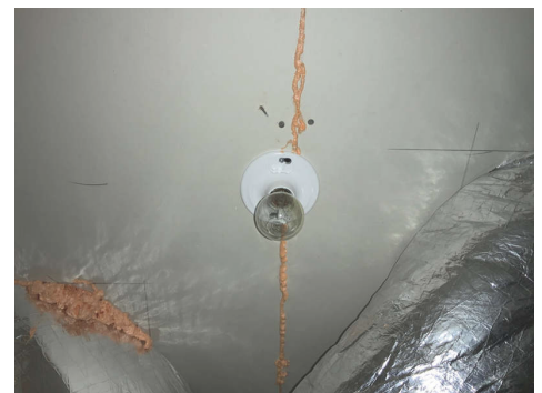
Utility Coset Garage
