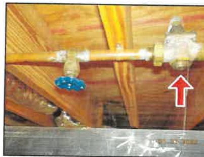
Adjustment/replacement of the pressure regulator valve (PRV) is necessary.
