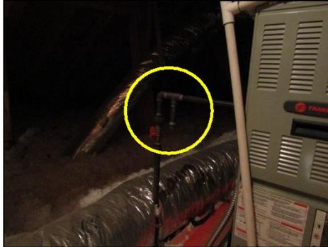
Attic HVAC: Improper sediment trap. Sediment present but not functional in its current installation. Sediment traps do as name notes, they trap sediment before it enter water heaters or HVAC systems and help prolong life. Recommend correction by qualified HVAC contractor.
