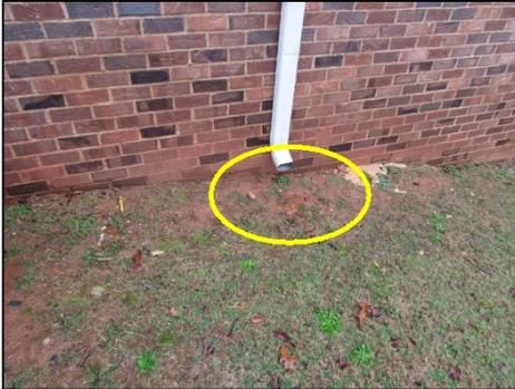
Extensions / Splash blocks missing or insufficient: Install to divert water away from the foundation.
