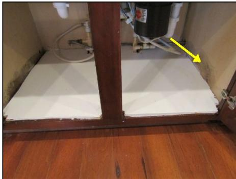
Signs of previous repairs noted under kitchen sink. No evidence of current leaks but slightly elevated moisture readings. Recommend review by a qualified contractor
