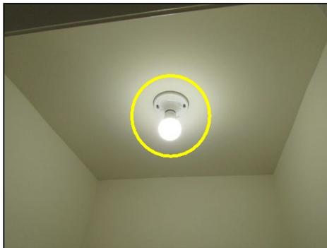
FIRE HAZARD: No globe at basement closet lights. This can cause a fire should stored items come in contact with a hot bulb. Recommend install globe or install new fixture by qualified electrical contractor.
