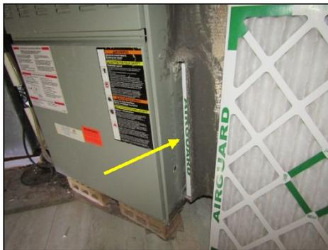
Filter covers missing. Recommend purchasing covers or keeping sealed with HVAC tape for proper functionality.
