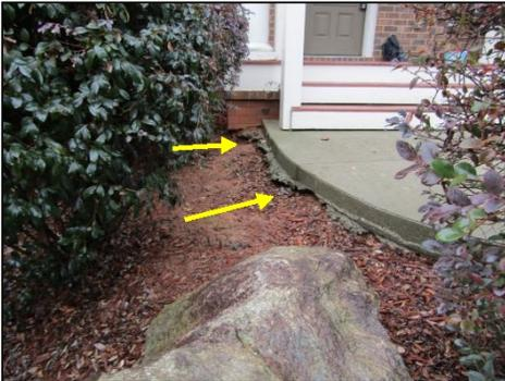
Erosion noted in some areas. Recommend review by a qualified contractor to prevent erosion and cracking of slabs or deck footings.
