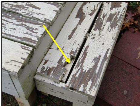
Step tread is loose/damaged. Safety concern. Recommend review for repair by a qualified contractor.
