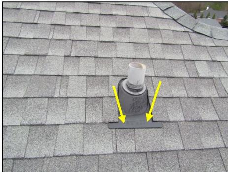
Missing nails at vent cap. Nails are needed for proper fastening. Recommend review by a qualified contractor.
