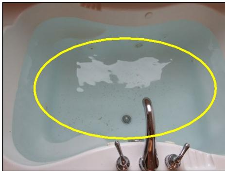
Debris was ejected from the jets during operation. Recommend sanitary flush to clean jets.
