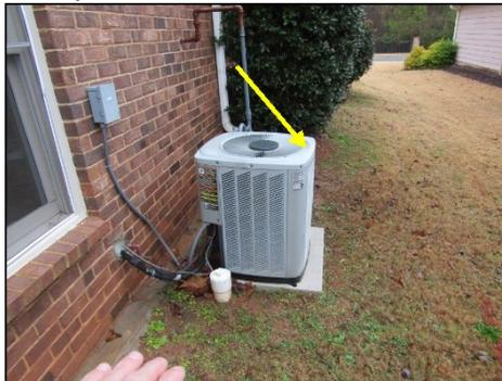
Left side AC compressor not level. When a compressor is out-of-level, the oil can separate and the compressor may operate without adequate lubrication. Recommend review and adjustment by qualified HVAC contractor.
