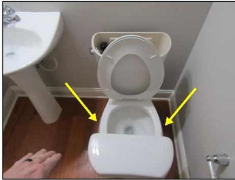
Multiple toilet bowls loose. The wax ring inside the unit must have a snug, secure fit in order to keep from leaking. Recommend repair by qualified plumbing contractor.
