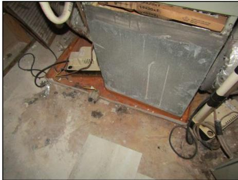
Heater base functional at time of inspection. Tub indicates previous leakage. Monitor and consult with previous owners for explanation.
