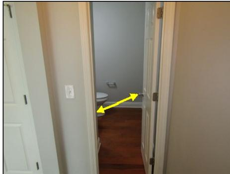
Some doors do not latch correctly. Recommend adjustment to door and/or striker plate by qualified contractor.
