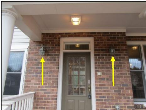
Light switch damaged or bulb inoperable. Recommend replacing bulbs and reviewing with seller prior to close to ensure it will not require professional repairs.
