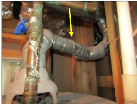
SAFETY CONCERN: The vent pipe from the natural draft gas water heater fails to rise 1/4" per foot. This can prevent the carbon monoxide from properly leaving the home. In the interest of safety, recommend review and repair by qualified HVAC contractor.
