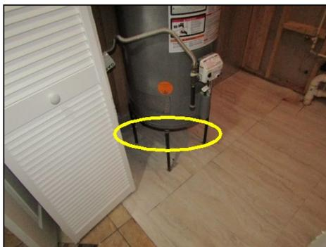
No overflow pan noted. While not required in unfinished slab areas, pan is suggested when finished area can be affected by leakage of the water heater. Recommend review or installing by qualified plumbing contractor.
