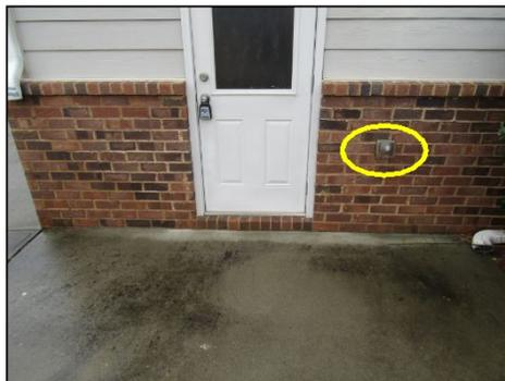
Outlet at right side of garage is not GFCI protected. In the interest of safety, locations such as garages, unfinished basements, kitchens, laundry rooms, outside area and all plumbing fixtures within 6 feet should be GFCI protected. Recommend review by qualified electrical contractor.
