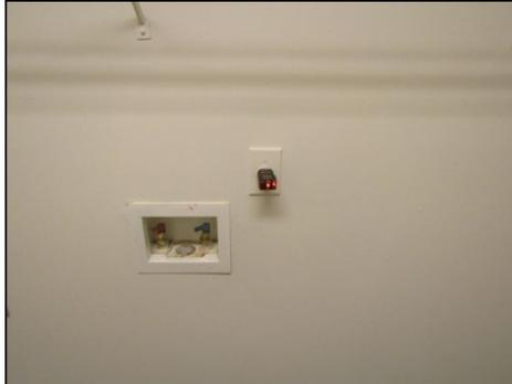
Outlet is not GFCI protected. While this was not a common building practice when the home was constructed, In the interest of safety, locations such as garages, unfinished basements, kitchens, laundry rooms, outside area and all plumbing fixtures within 6 feet should be GFCI protected. Recommend review by qualified electrical contractor.
