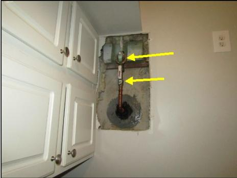
Pressure regulator and main water shut off located in cutout at front of home in basement wall.
