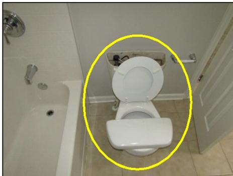
Jack and jill toilet was not functional at time of inspection. Toilet was empty and evidence of prior moisture at wall behind toilet may indicate a leak. Recommend review by a qualified plumbing contractor.
