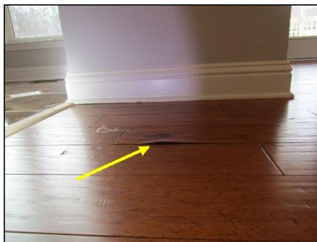
Hardwood floor in one area of dining room is lifting. No evidence of moisture intrusion. Recommend review by a qualified contractor.
