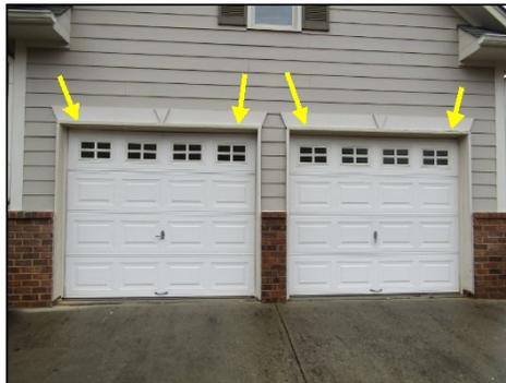
Flashing does not completely cover the trim at garage doors. This is a moisture concern. Recommend review/repair by a qualified contractor.
