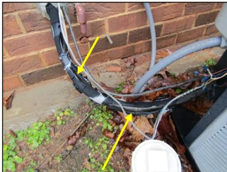
Insulation is deteriorated at refrigerant lines. This may effect the efficiency of unit. Recommend repairing or replacing by qualified HVAC contractor.
