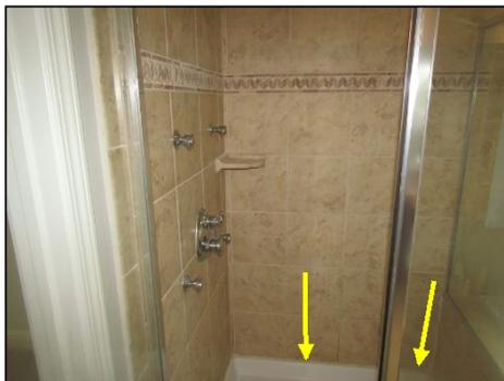
Missing grout and or caulk noted in master shower wall. This may allow moisture to penetrate walls and subfloor. Recommend review and repair by qualified contractor.
