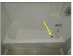
Tub functioned properly but drain stopper missing or not operational. Could not test overflow at time of inspection.
