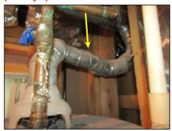
SAFETY CONCERN: The vent pipe from the natural draft gas water heater fails to rise 1/4" per foot. This can prevent the carbon monoxide from properly leaving the home. In the interest of safety, recommend review and repair by qualified HVAC contractor.
