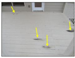
Staining bleeding through paint at deck. Typically connected. Recommend installing simpson ties by this is caused when paint is applied over saturated wood. Recommend review by a qualified contractor.
