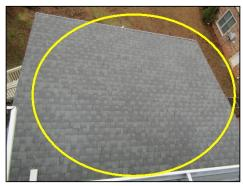
Patio roof has asphalt shingles installed on a slope of less than 2/12. Generally, this is not recommended as moisture can seep under the shingles and makes the shingles more prone to wind damage. Recommend review by a qualified roofing contractor.
