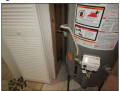
\* Proper Sediment trap noted on gas line.
