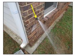
Left side of home: Faucet not sealed or secure to siding. Possible damage to supply line or moisture intrusion. Recommend repair by qualified contractor.
