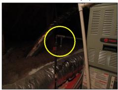
Attic HVAC: Improper sediment trap. Sediment present but not functional in its current installation. Sediment traps do as name notes, they trap sediment before it enter water heaters or HVAC systems and help prolong life. Recommend correction by qualified HVAC contractor.
