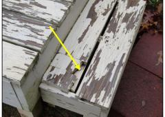
Step tread is loose/damaged. Safety concern. Recommend review for repair by a qualified contractor.
