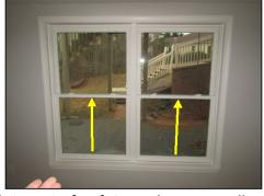
In the interest of safety and egress, all windows should be operational. At the time of the inspection, some windows were stuck closed. Recommend repair by a qualified contractor.
