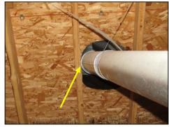
SAFETY CONCERN: Vent pipe is in direct contact with the roofing materials in attic. Note: Minimum furnace/water heater double wall vent pipe clearance from combustible material is 1". In the interest of safety, Recommend review for repair by qualified contractor.
