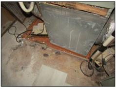
inspection. Tub indicates previous leakage. Monitor and explanation.
