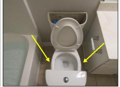
Multiple toilet bowls loose. The wax ring inside the unit must keep from leaking. Recommend repair by qualified plumbing contractor.
