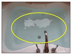
Debris was ejected from the jets during operation. Recommend sanitary flush to clean jets.
