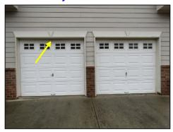
Damage noted at the top of the left side garage door. Recommend review or repair by qualified garage door contractor for proper functionality.
