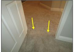
Carpet is loose and rolling in Recommend review and repair by a qualified flooring contractor. by a qualified flooring contractor.
