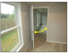
Some doors do not latch correctly. Recommend plate by qualified contractor.
