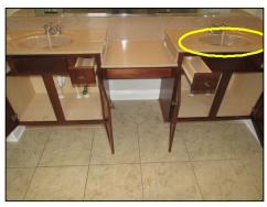
Slow drain at right side master sink, indicates drain line needs cleaning and/or drain not properly vented. Recommend review and repair by qualified plumbing contractor.
