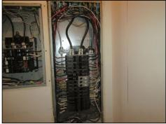
No major system or function concerns noted at Improper clearance from panel front. 30 inches time of inspection at main or subpanel box except side to side is recommended. Recommend adding where noted.
