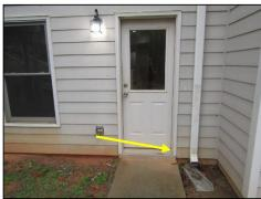
Moisture damage/wood rot noted Left side, basement exterior door at back door casing. Recommend review or repair by Recommend adjustment of the qualified contractor.
