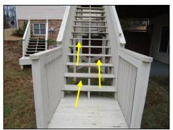
Stairs missing step risers. For the interest of safety, recommend step riser have no more than 4" of gap. Recommend review and repair by qualified general contractor.
