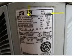
Compressor unit is a 3 1/2 ton system manufactured in 2006. National average designed life expectancy of AC unit is 10-12 years. Budget for possible repair or replacement in the near future.
