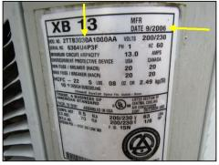
Compressor unit is a 2 1/2 ton system manufactured in 2006. National average designed life expectancy of AC unit is 10-12 years. Budget for possible repair or replacement in the near future.
