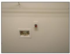
Outlet is not GFCI protected. While this was not a common building practice when the home was constructed, In the interest of safety, locations such as garages, unfinished basements, kitchens, laundry rooms, outside area and all plumbing fixtures within 6 feet should be GFCI protected.
