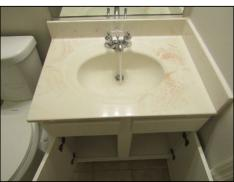
Faucet functioned properly but drain stopper missing or not operational.
