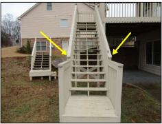
Some handrails are loose with lag bolts missing from handrail supports. It is recommend at least 2 bolts are installed to ensure the rails are secure. In the interest of safety, recommend review/repair by a qualified contractor.
