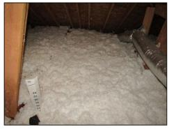
Insulation depth is less than 13 inches in some review and repair by a professional Pest or wildlife areas. Recommend adding insulation to achieve a consistent R-30 Value/ or 13+ inches for energy efficiency.
