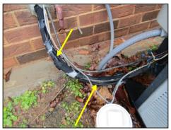
Insulation is deteriorated at refrigerant lines. This may effect the efficiency of unit. Recommend repairing or replacing by qualified HVAC contractor.
