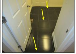
Cracking or popping ceramic tiles. This is an indication of inadequate subfloor installation. Recommend review and repair by qualified flooring contractor.
