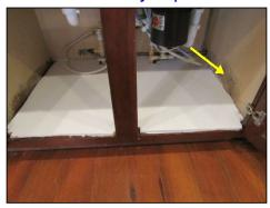
Signs of previous repairs noted under kitchen sink. No evidence of current leaks but slightly elevated moisture readings. Recommend review by a qualified contractor
