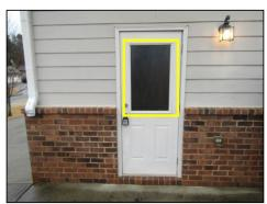
Fog/condensation observed in exterior garage door window. This indicates a failed seal. This reduces the energy efficiency of the window. Recommend review by a qualified contractor.
