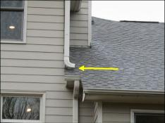
Downspouts terminate perpendicular to the roof shingles. This can allow water to flow under the shingles and lead to roof leaks. Recommend repair by a qualified gutter contractor.
