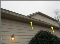
Peeling paint, damaged trim, split caulk, and exposed wood noted and should be addressed for repairs to prevent moisture damage. Recommend full review damage. Recommend full review damage. Recommend full review and repair of homes paintable areas.
