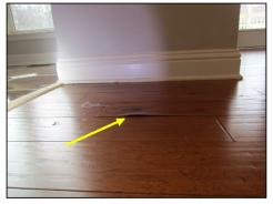
Hardwood floor in one area of dining room is lifting. No evidence of moisture intrusion. Recommend review by a qualified contractor.
