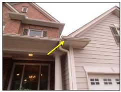
Peeling paint, damaged trim. split caulk, and exposed wood noted and should be addressed for repairs to prevent moisture and repair of homes paintable areas.
