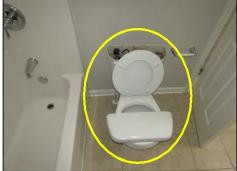
Jack and jill toilet was not functional at time of inspection. prior moisture at wall behind toilet may indicate a leak. Recommend review by a qualified plumbing contractor.
