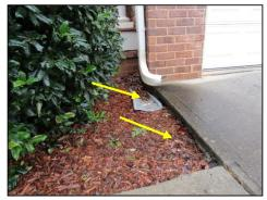
Erosion noted in some areas. Recommend review by a qualified contractor to prevent erosion review by a qualified contractor to prevent erosion and cracking of slabs or deck footings.
