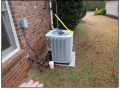
Left side AC compressor not level. When a compressor is outof-level, the oil can separate and the compressor may operate without adequate lubrication. Recommend review and adjustment by qualified HVAC
