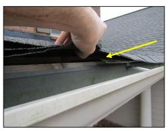
No drip edge flashing noted leaving underlying framing exposed to weather. While this was not a standard building practice at the time the home was constructed it is a recommended current standard. Recommend review by qualified roofing contractor.
