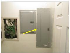
Missing screw in panel cover. Recommend installing the approved screw by a qualified contractor.
