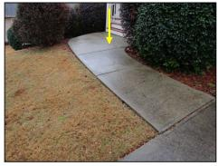
Sidewalk in good condition. Common settlement cracks noted. Recommend sealing to prevent further expansion.
