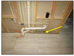
Active leak noted at basement kitchenette sink. Recommend repair by a qualified plumbing contractor to prevent moisture damage.
