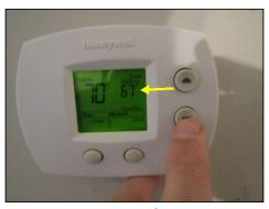
Functional at the time of inspection but the upstairs and the main level thermostat temperature would not go below 67 F when the air temperature would not go below 67 F when the air was on. This may be programmed stop.
