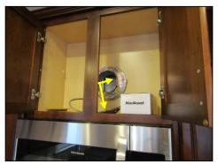
Vent functioned but exhaust vent was not connected to exterior venting. In order for the vent to function properly a pipe should be connected. Recommend review and repair by a qualified contractor.
