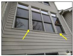
repairs to prevent moisture damage. Recommend repairs to prevent moisture damage. Recommend full review and repair of homes paintable areas.
