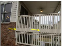
Some handrails are loose with lag bolts missing from handrail supports. It is recommend at least 2 bolts are installed to ensure the rails are secure. In the interest of safety, recommend review/repair by a qualified contractor.
