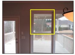
Cloudiness/condensation observed in double pane window. This is an indication of a failed seal. Recommend review by qualified contractor.
