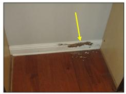
Termite activity noted in the kitchen. Recommend review by a qualified termite and pest control contactor.
