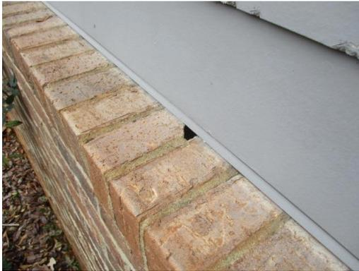
Small opening noted in the brick work at the right side of the detached garage area; tuck pointing or sealing is recommended.
