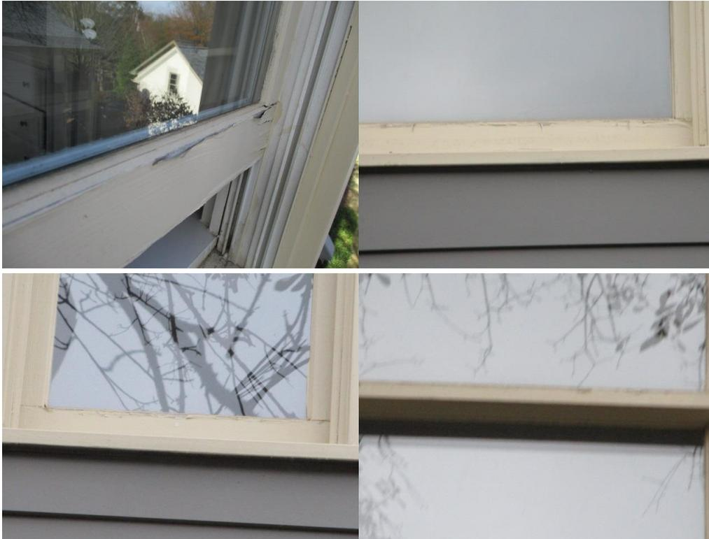
Failing and peeling paint noted on windows around the home particularly in the bottom rails.
