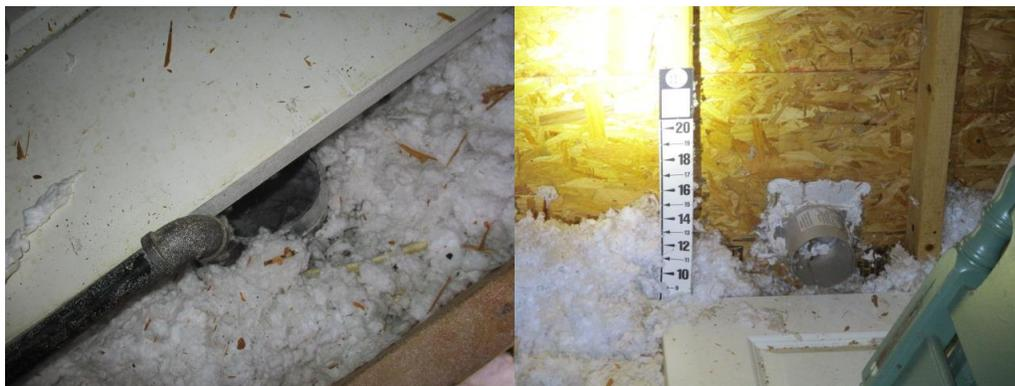
It appears the dryer vent has been redirected with abandoned sections noted in the attic space.
