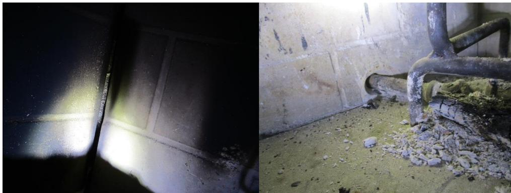
Openings were noted in the refractory panels in the fireplace at the rear corner and at the gas supply entry.
