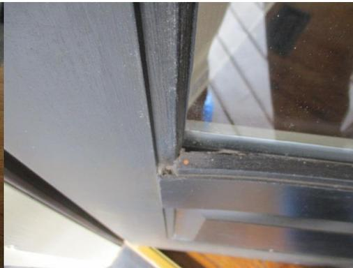
Lost seal noted in the window unit of the front door with some swelling noted in the enclosure.
