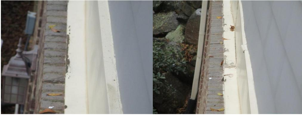
Localized rot and failing paint noted in the wood transition trim at the right side exterior.
