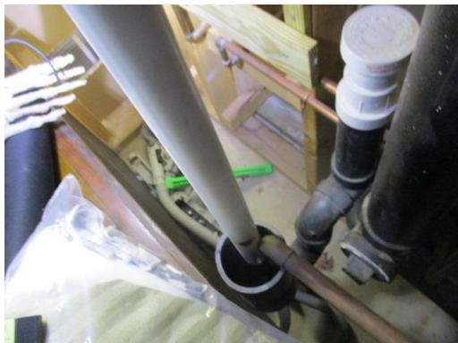
An open trap was noted at the basement mechanical area for discharge lines with no apparent way to consistently prime the trap. A plumber should be consulted to install a trap primer or trap fixture fitting.
