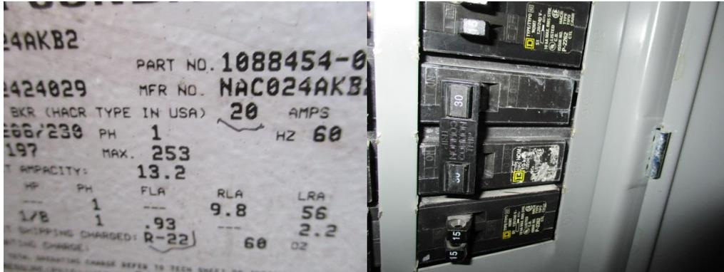
The air conditioning systems were noted to be older with listing for R22. The comfort maker unit was noted to be listed for a maximum over current protection of 20 amps with a 30 amp breaker installed in the main panel.
