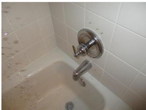
Missing handle noted at the basement bathroom tub enclosure fixture.
