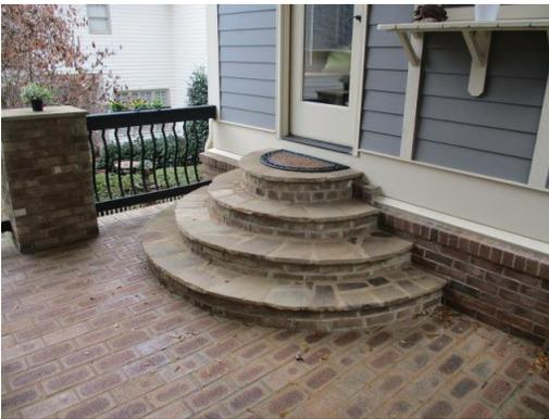
Steps noted to be lacking handrails at the front entry and both rear entry areas.
