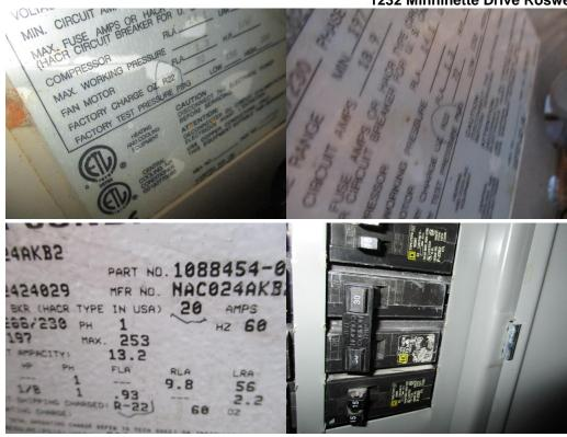
The air conditioning systems were noted to be older with listing for R22. The comfort maker unit was noted to be listed for a maximum over current protection of 20 amps with a 30 amp breaker installed in the main panel.
