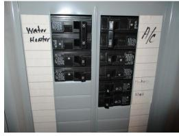
The subpanel serving the detached garage and loft area lacks full labeling and AFCI protected breakers for sleeping areas.
