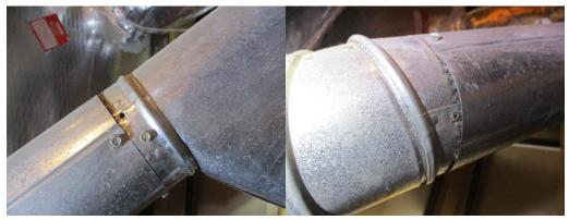
The 1<sup>st</sup> picture illustrates improper installation of venting with the lower section over the top section which can cause leakage. The 2<sup>nd</sup> picture shows the beginning of the transition that was likely altered at water heater replacement. The fittings should be properly attached and sealed as needed to prevent leakage of exhaust gases.
