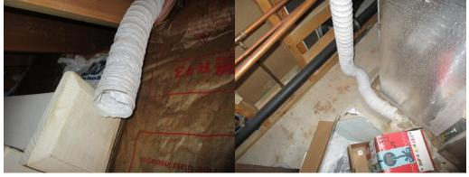
Bathroom exhaust fan vents were noted to lack termination to the building exterior at the detached garage area walk in knee wall attic space and at the basement mechanical area.
