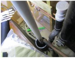
An open trap was noted at the basement mechanical area for discharge lines with no apparent way to consistently prime the trap. A plumber should be consulted to install a trap primer or trap fixture fitting.
