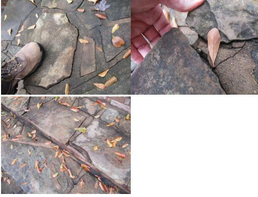
Loose and damaged stone treads noted at the front entry steps.
