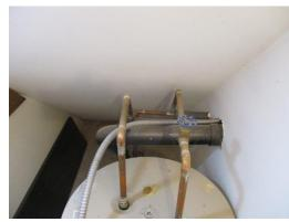
The circuit serving the water heater unit at the detached garage area was noted to lack the required electrical service disconnected.
