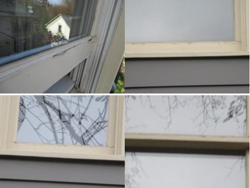
Failing and peeling paint noted on windows around the home particularly in the bottom rails.
