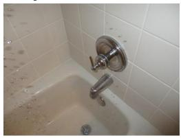
Missing handle noted at the basement bathroom tub enclosure fixture.
