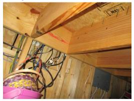
The support joists below the basement stairwell landing were noted to lack end bearing.
