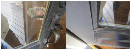
Lost seal noted in the window unit of the front door with some swelling noted in the enclosure.
