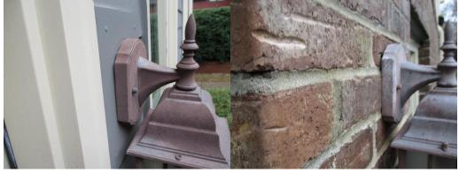
Loose light fixture noted at the rear exterior and right side exterior; recommend securing and sealing.
