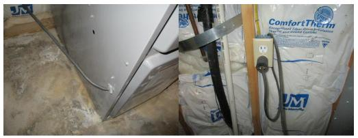
Amateur wiring was noted at the comfort maker furnace in the basement area. The unit lacks hard wiring with an available service switch.
