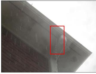
4.3 Item 3(Picture) Leaking gutter, above garage
