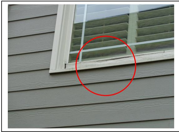
Moisture damage to exterior surface of master bath window.
