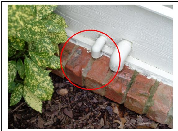
Water flowing from pressure relief drain at left side of home.
