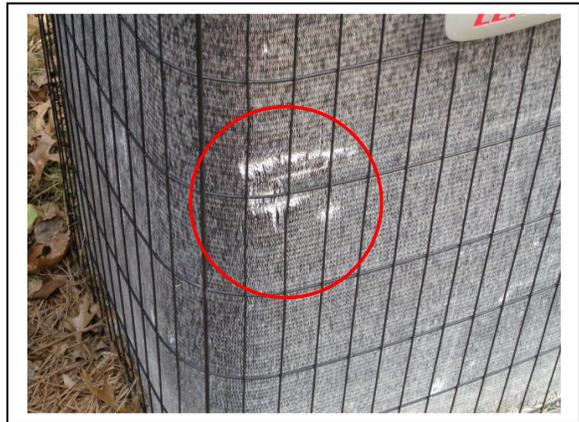
Damaged cooling fins at front exterior A/C unit.
