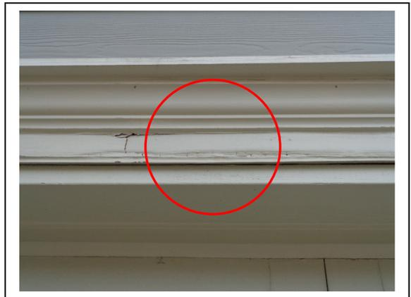
Moisture damage to exterior trim above garage door opening.
