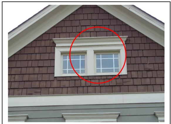
Possible moisture damage to exterior front window surfaces.
