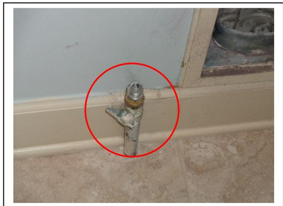
Gas pipe at upstairs laundry room is missing cap.
