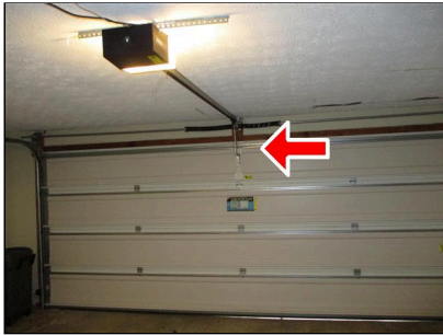
4.7 DOOR OPERATOR(S) (Picture 1) No reverse
