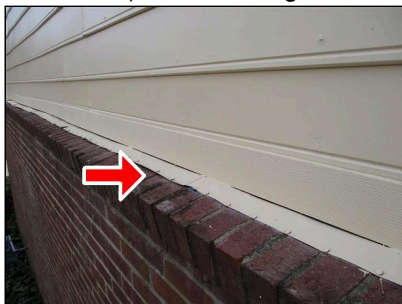
3.2(2) EXPOSED FLASHING (Picture 1) Nailed flashing
