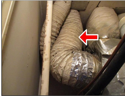
11.6 DISTRIBUTION SYSTEM (Picture 1) No insulation
