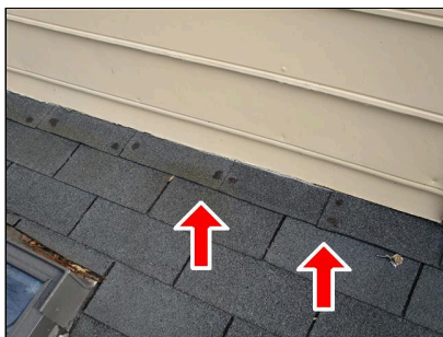
3.0 ROOF COVERING (Picture 1) Worn sealant
