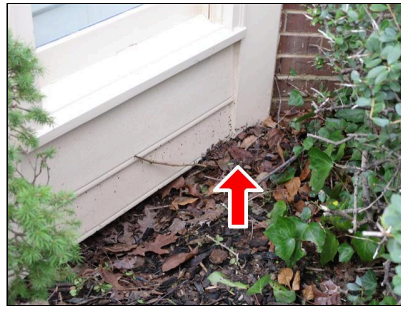
1.1 SIDING 2 (Picture 1) Wood/ground contact
