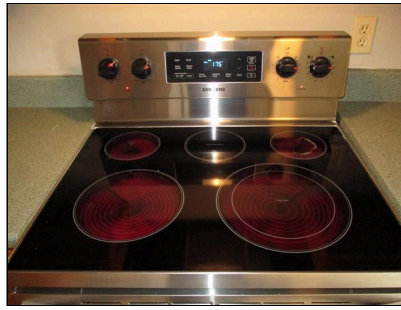
7.4(2) RANGE (Picture 1) No tip over protection
