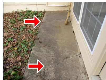
2.0(2) WALKWAYS (Picture 1) Settlement cracking
