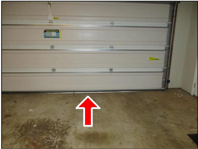
4.6 VEHICLE DOOR(S) (Picture 1) Daylight at door
