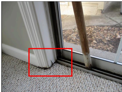
1.4 ENTRY DOORS (Picture 2) Water intrusion
