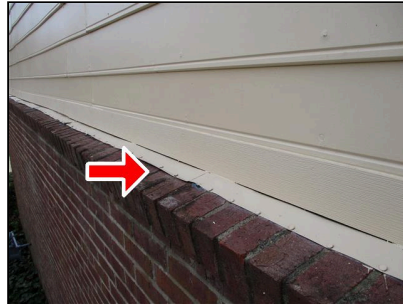
Nailed flashing
