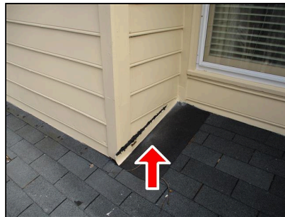
Check flashing
