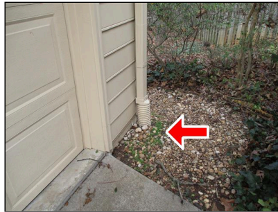
3.7(2) DOWNSPOUTS / ROOF DRAINS (Picture 1) Ground drain
