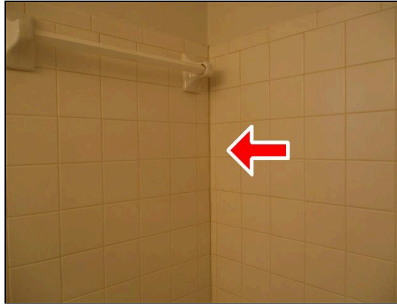
6.21 WALL TILE (Picture 1) Seal as needed
