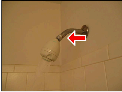
6.20 BATHTUB (Picture 1) Leaking
