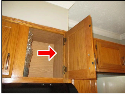
7.8 CABINETRY (Picture 1) Loose hinges
