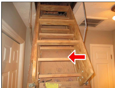
5.4(1) ATTIC STAIRS (Picture 1) Add insulation
