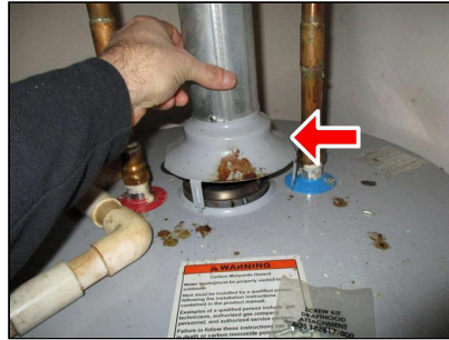
14.2 (Picture 1) Loose diverter
