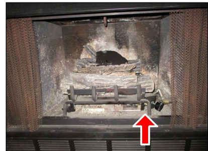
8.9 FIREPLACE (Picture 1) No gas/pilot/knob inoperable
