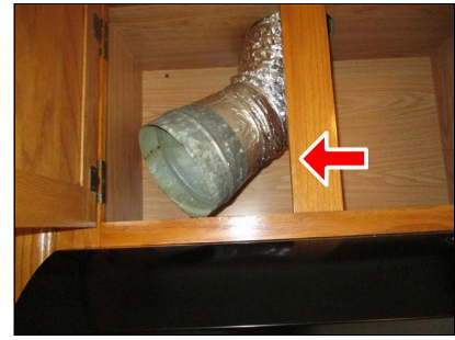
7.7 VENTILATOR (Picture 1) Loose vent
