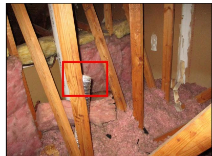
6.14 VENTILATOR (Picture 1) Bathroom vent
