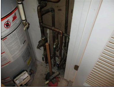
PRV/water cut-off
