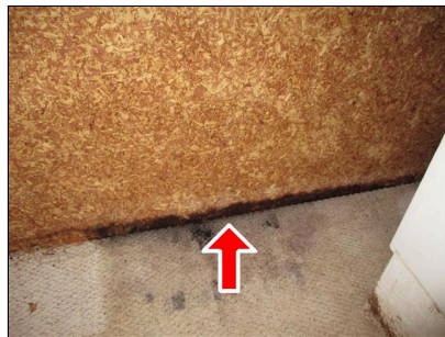
9.1 (Picture 1) Water intrusion
