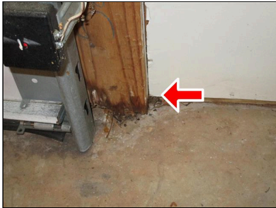
4.1 EXPOSED FRAMING (Picture 1) Water staining
