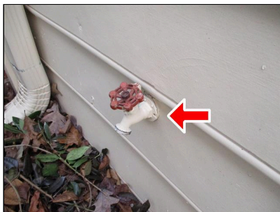
1.8 EXTERIOR FAUCET(S) (Picture 1) Add backflow preventer
