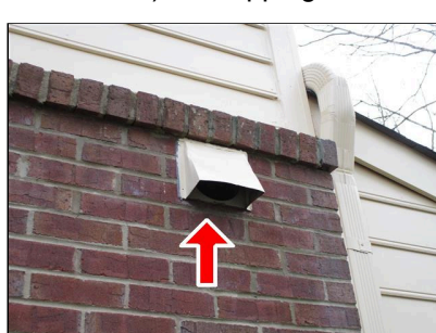
1.9 EXTERNAL VENTS (Picture 1) No screen
