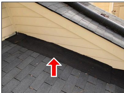
3.2(1) EXPOSED FLASHING (Picture 1) Improper flashing
