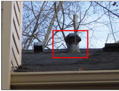
3.4(2) VENTILATION COVERS (Picture 1) Unused vent
