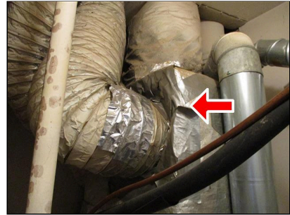
11.6 DISTRIBUTION SYSTEM (Picture 2) Incorrect tape
