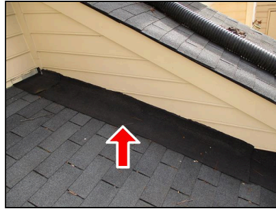
Improper flashing
