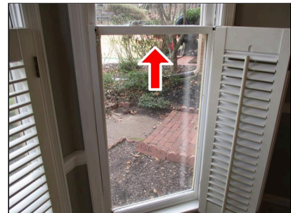
8.5(2) REPRESENTATIVE WINDOWS (Picture 3) Stuck window
