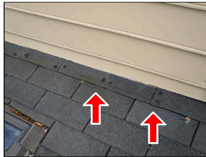
3.0 (Picture 1) Worn sealant
