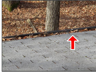
3.6 (Picture 2) Missing screen
