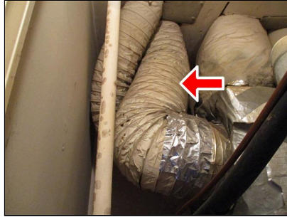
11.6 (Picture 1) No insulation
