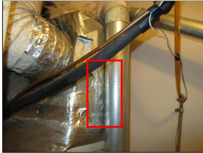
11.4 VENT CONNECTOR 1 (Picture 1) No clearance
