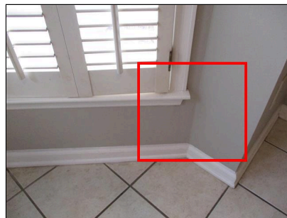
8.1 (Picture 1) Water intrusion
