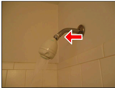
6.20 (Picture 1) Leaking
