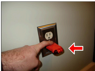
6.6 ELECTRIC / GFCI (Picture 1) No GFCI
