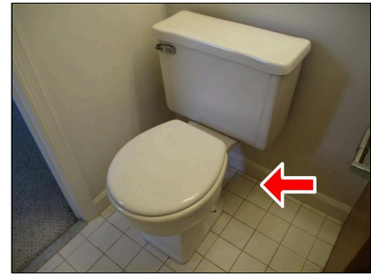
6.19 TOILET (Picture 1) Loose at floor
