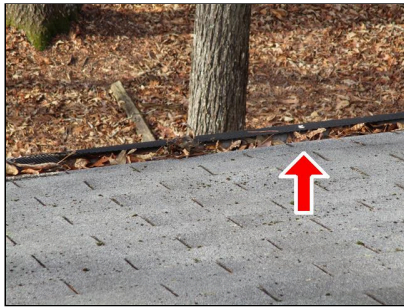
3.6 RAIN GUTTERS / EAVESTROUGHS (Picture 2) Missing screen
