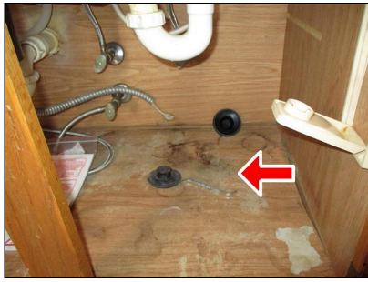
7.0 PLUMBING / SINK (Picture 1) Prior staining
