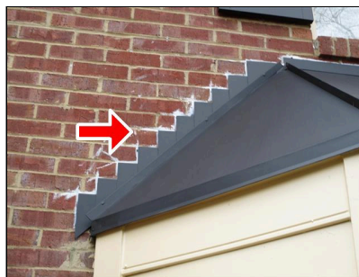
3.1 ROOF COVERING 2 (Picture 2) Not sealed
