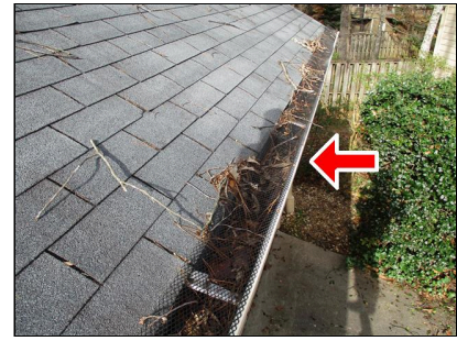
3.6 RAIN GUTTERS / EAVESTROUGHS (Picture 1) Clean gutters
