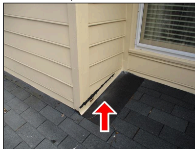
3.2(3) EXPOSED FLASHING (Picture 1) Check flashing
