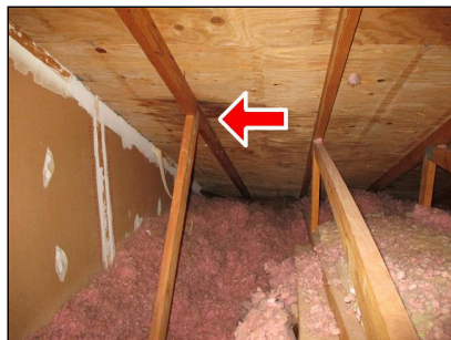
5.1(2) ROOF DECK / SHEATHING (Picture 1) Prior staining
