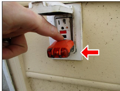
1.7 ELECTRIC / GFCI(S) (Picture 1) Not tripping
