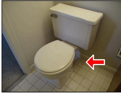
6.19 (Picture 1) Loose at floor
