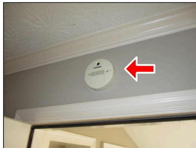
8.8(2) DETECTOR ALARM TEST (Picture 1) Expired detector
