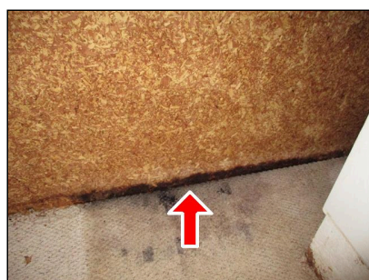
9.1 HOUSE FLOOR SLAB (Picture 1) Water intrusion
