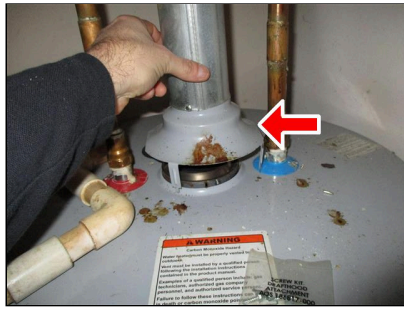
14.2 VENT CONNECTOR (Picture 1) Loose diverter
