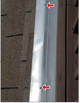
(2) There are uplifted shingles on the right side of the house. A qualified roofer needs to re-nail shingles and seal any holes with a roofing sealant as needed.
