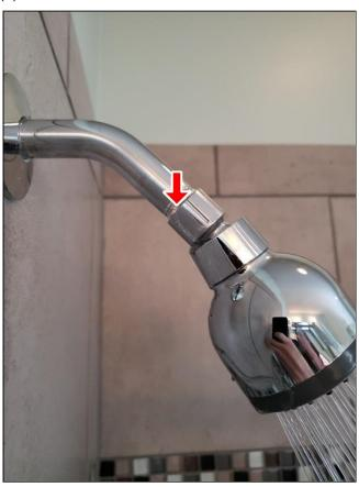
(3) Water pressure drops in the master bath and hall bath when more than one plumbing fixtures is turned on. A licensed plumbing contractor needs to repair.
