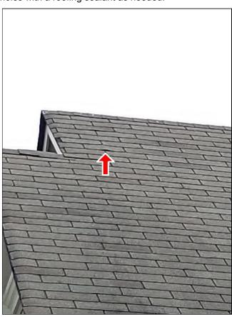
(3) There are uplifted or wind blown shingles on the back of the house. A qualified roofer needs to inspect further and repair.
