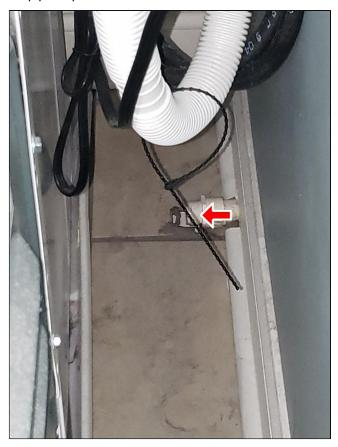
(2) The washer hoses are not stainless steel braided hoses. Recommend using stainless steel braided washer hoses to connect washing machine. Stainless steel braided hoses last about 5 years. The black hoses only last about 3 years.
