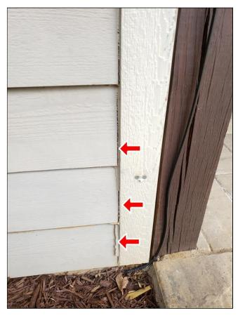
(3) Corner boards on the chimney need to be caulked and painted. A qualified contractor needs to repair.
