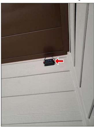
(2) The exterior light fixture at the front door and back door did not turn on. Replace bulb and verify operation of light fixture. In the event the light fixture does not work, a licensed electrician needs to repair.
