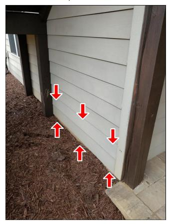
(2) The siding joints/ends needs to be caulked on the back of the house. See pictures for examples. A qualified contractor needs to caulk siding and paint to match existing as needed.
