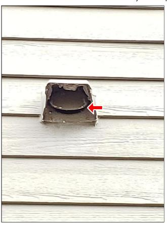
(2) The dryer duct pipe needs to be cleaned out from duct termination back to the dryer. Dryer duct pipe needs to be cleaned out every year. A qualified contractor needs to repair. 8.2 Insulation In Attic
