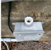
Stephanie, ¿- I stopped by the entrance this morning. ¿- It looks like a Handyman installed your box. ¿\* No ground rod & no cover and no plug on a hot line going to your sprinklers timmer. ¿\* The way it is very dangerous & sure doesn't meet code. ¿\* Between appointments I'll text you on replacing your 2 damaged spot lights. ¿Thanks, ¿Gary
