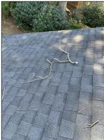
4. <u>SERVICE / REPAIR:</u> Improper sealant noted at ridge. Foam is not a exterior approved sealant. Recommend professional roofing contractor repair.
