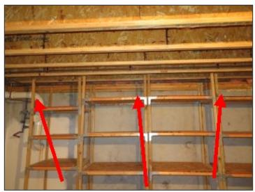
Foundation anchors not secured to sill plate
