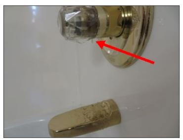
Active leak at handle valve in upstairs bathroom tub
