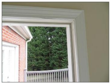
Missing weatherstripping at rear deck entry door
