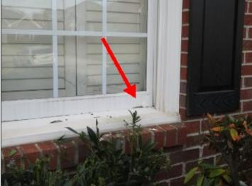
Damaged window frame at front left garage window
