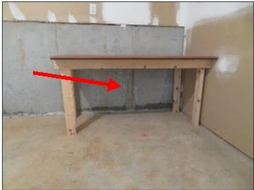
Evidence of water entry at plumbing drain line Evidence of water entry at side foundation wall penetration in garage
