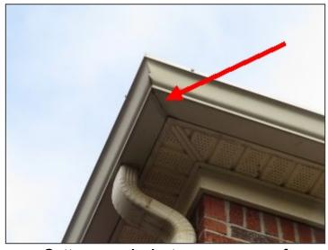
Gutter seam leak at rear corner roof
