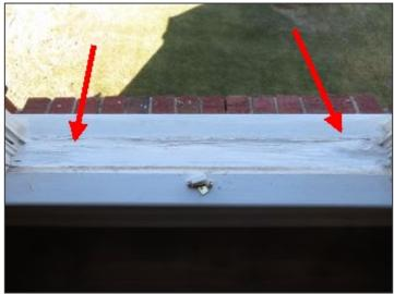
Damaged window sill at front bonus room window
