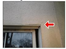
1.0(2) SIDING (Picture 3) Deterioration/water penetration
