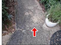
2.1 WALKWAYS (Picture 1) Settlement cracking
