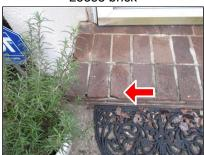
1.3 STAIRS / STOOPS (Picture 2) Settlement cracking
