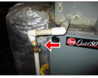
9.4 CONDENSATE PROVISIONS1 (Picture 1) No air gap/clamp at line
