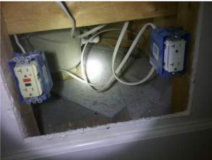
**86:** Outlets near hydro pump motor are missing cover plates
