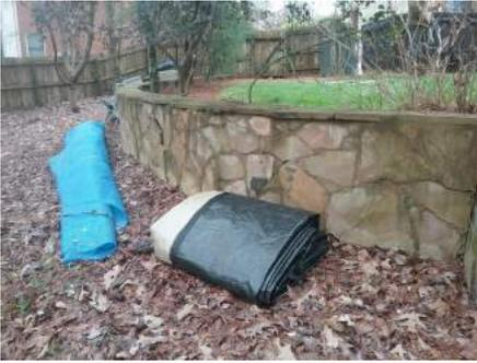
**43:** Settlement displacement/Cracks noted. Monitor in future years and budget to replace depending on the movement over the next few years.
