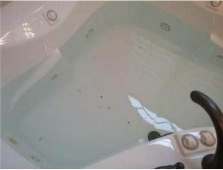
**85:** No access to tub jet motor. Without access to the tub jets repairs will be difficult.
