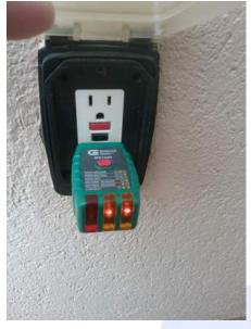
**123:** Recommend GFCI outlets be installed in kitchen outlets. While a homeowner is not required to upgrade older outlets, pre 1991 to GFCI protection we recommend all outlets in potentially wet areas be updated to increase safety for all occupants.
