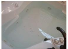
85: No access to tub jet motor. Without access to the tub jets repairs will be difficult.
