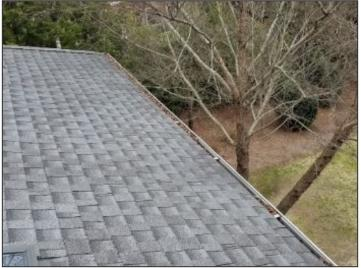
Gutter debris at rear roof
