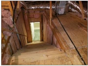
No guard railing at top of attic staircase
