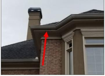
Damaged fascia at left side master bathroom roof
