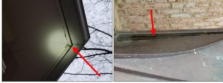
Gutter seam leak at rear deck roof
