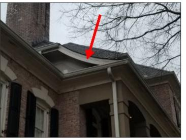
Damaged soffit at front left corner roof
