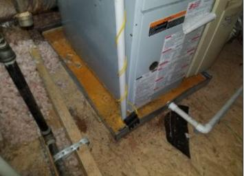
Rust staining in drain pan below master furnace
