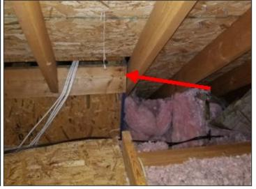
Evidence of a previous leak at corner of family room chimney - dry at time of inspection
