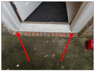
Damaged wood trim at basement entry door
