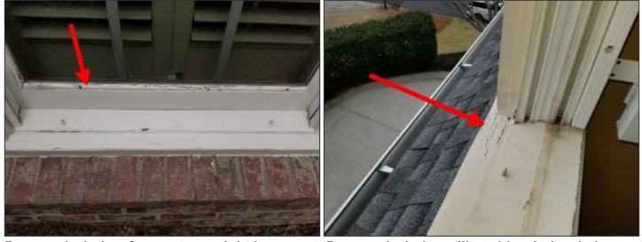
Damaged window frame at rear right basement Damaged window sill at side window in bonus window room above garage
