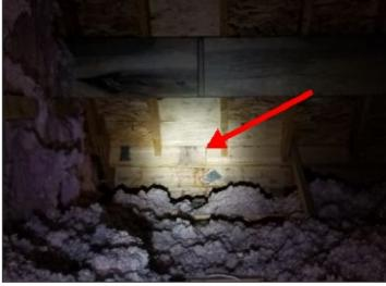
Evidence of an old leak at front roof above office
