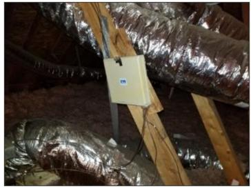
Dual zone thermostat control for second floor HVAC system
