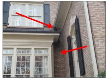
Water staining at dining room brick wall below gutter
