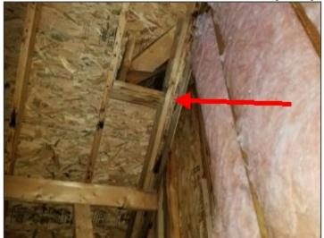
Evidence of a previous leak at rear roof intersection behind family room chimney
