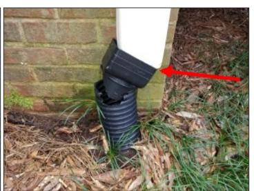
Disconnected downspout at left garage corner
