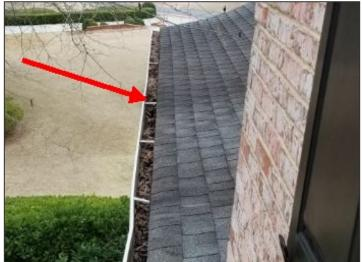
Gutter debris at front roof
