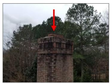
Missing flue caps at masonry chimneys
