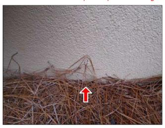
(2) Deterioration and/or swelling observed in sections of the hardboard siding located at the left side of the home. This material is subject to water absorption and should be regularly painted/sealed to prevent moisture damage. Suggest further evaluation by a qualified contractor for maintenance and/or repairs to prevent further damage/deterioration or replacement as needed.
