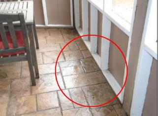
(2) The deck support posts are resting in concrete. This limits the inspectors ability to determine proper footings under the posts, limits the review of potential damage/deterioration at the base of the posts, and may cause wood deterioration/moisture damage. it is typically advised that support posts rest on cleats that allow air-flow around and under the posts. Recommend further evaluation for corrections as needed by a licensed contractor prior to close.
