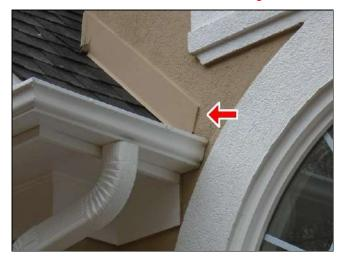
(2) Inspector is unable to determine if step flashing is present. Visible flashing observed installed over the shingles whereas step flashing is installed beneath the shingles. Recommend further evaluation by a licensed roofer to verify proper installation of the flashing or for corrections as needed prior to close.
