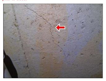
(2) Efflorescence is present on the front foundation wall in the basement at an area of cracking. Efflorescence is the salts left behind from moisture soaking into or passing through a masonry product. This moisture could adversely affect the foundation and/or the basement environment. Recommend review by a licensed contractor specializing in moisture control to determine the source of moisture and recommend or make necessary corrections to prevent further moisture intrusion.
