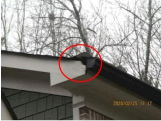
Exterior Surface: trim board damages
