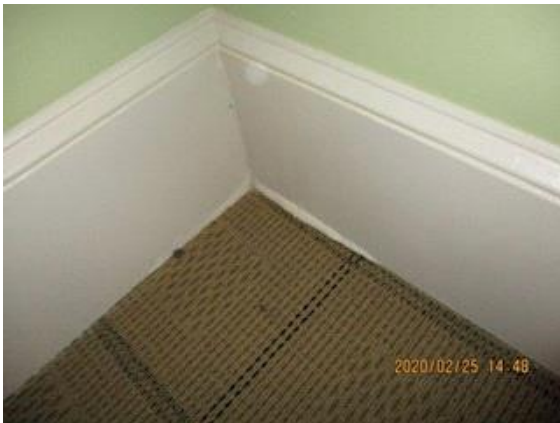
Basement grand room : baseboard water damages
