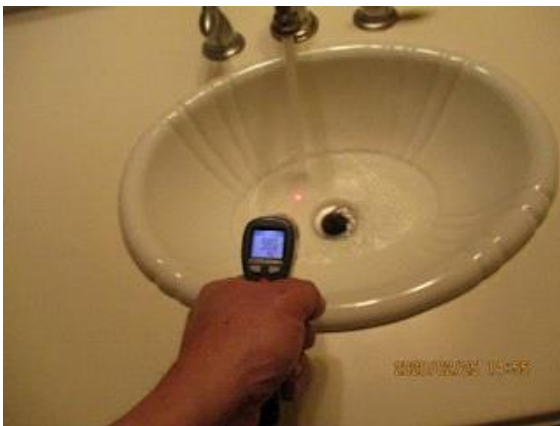
Basment full bathroom : Sink drainage stopper assembly missing
