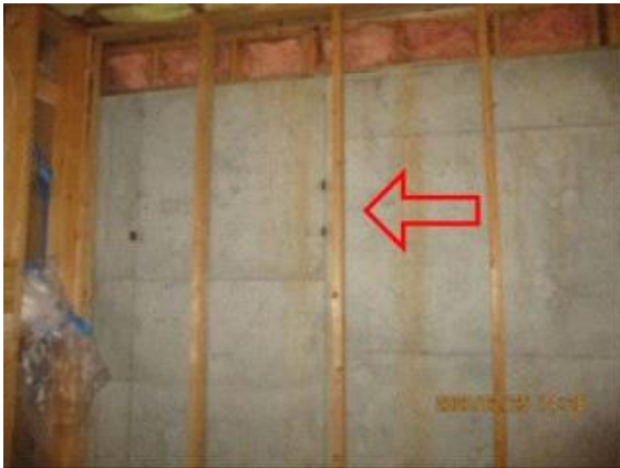
Interior Foundation: basement foundation wall cracks
