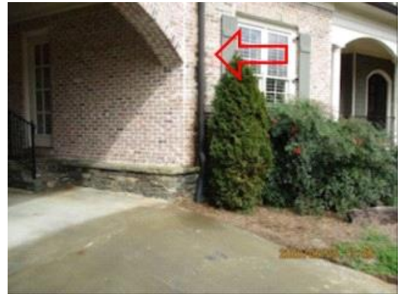
Gutters/Down Spouts: Gutter / downspout was overflowed and was leaking water
