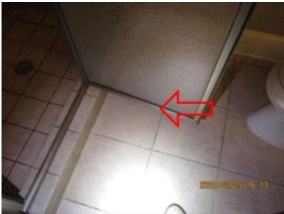
upper rear bathroom : Shower door rubber seal was torn / missing
