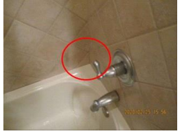
upper front left bathroom : Defective grout at the shower enclosure
