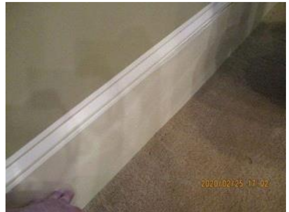
Basement grand room : water damages at the baseboard
