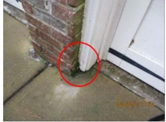
Garage/Carport: exterior wood trim rotten near the bottom
