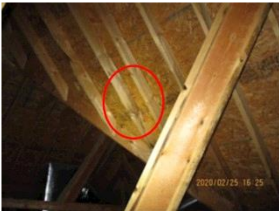
Attic Framing/Sheathing: Water stain on the attic deck
