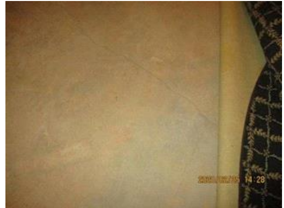
Floor/Slab: Basement floor cracks
