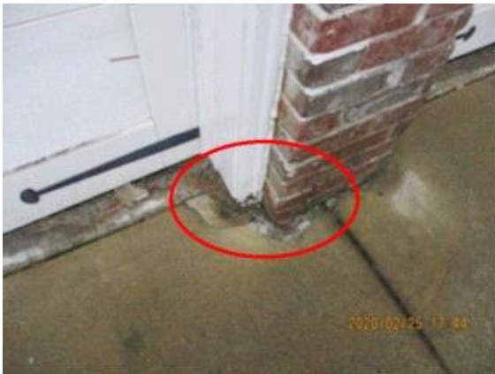
Garage/Carport: wood trim outside rotten near the bottom
