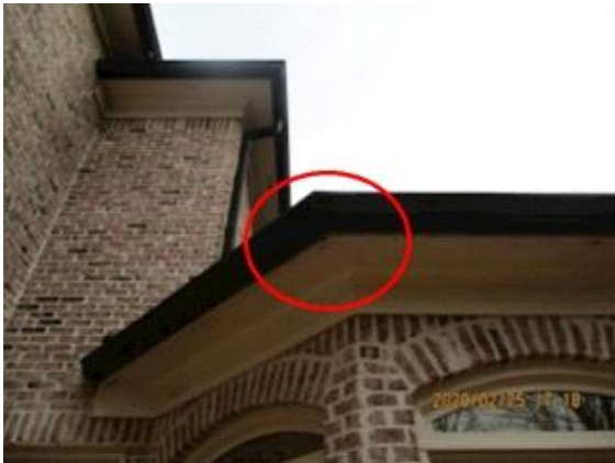
Gutter : gutter outside the kitchen leaking water at the seam
