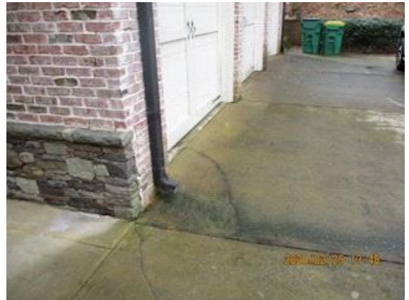
Driveway: cracked driveway surface
