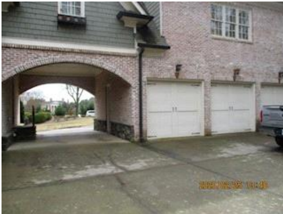
Driveway: cracked driveway surface
