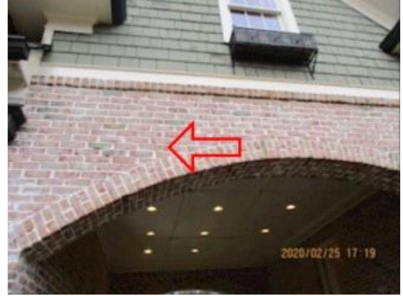
Exterior Surface: cracks on brick wall
