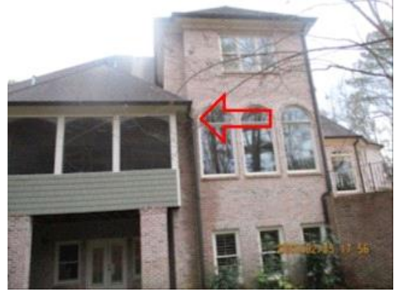
Gutters/Down Spouts: Gutter appear leaking water
