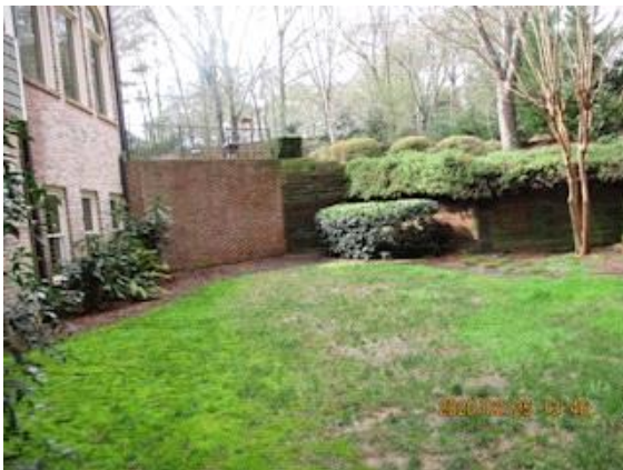
Grading / Drainage: Near level grading at the back of the property, may pose slow drainage problem, water ponding noticed
