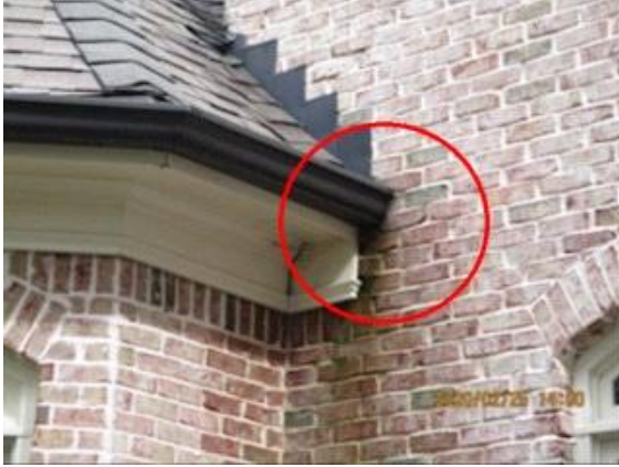
Gutters/Down Spouts: gutter leaking water at the end
