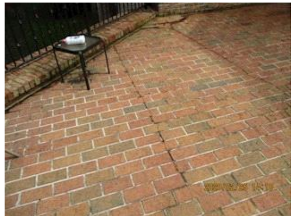
Patio: cracks and settlements
