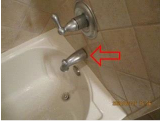
upper front left bathroom : bathtub spout need caulking
