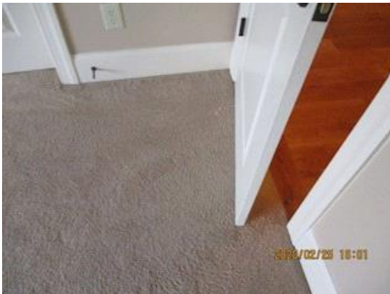
upstair front middle room : door dragging on carpet
