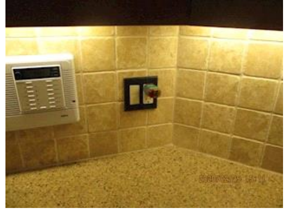
Kitchen @ main level : Electrical outlets at the countertop have no power
