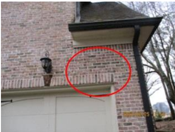
Exterior Surface: cracked brick wall
