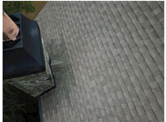
Roofing: previous roof repair behind the chimney
