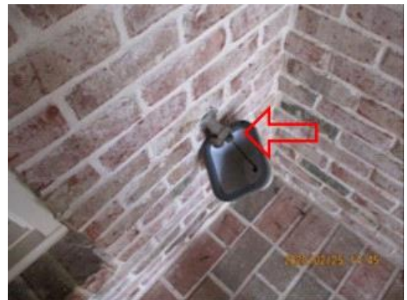
Exterior Surface: Basement exit faucet handle missing
