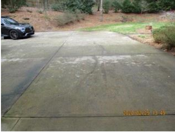
Driveway: cracked driveway surface
