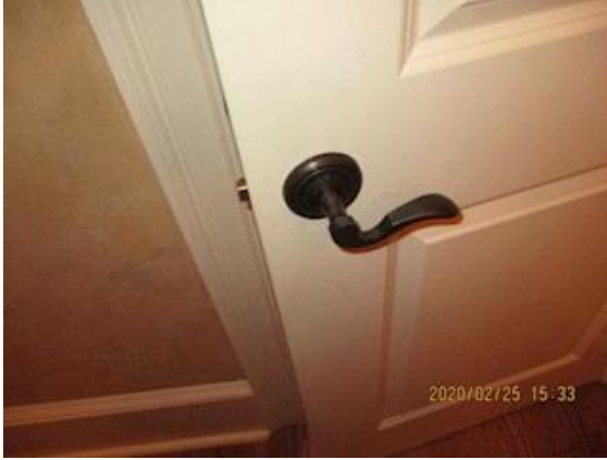
main level half bathroom : door missing a lock
