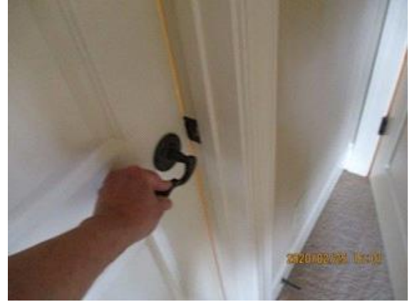
upstair front middle room : closet door could not engaged properly
