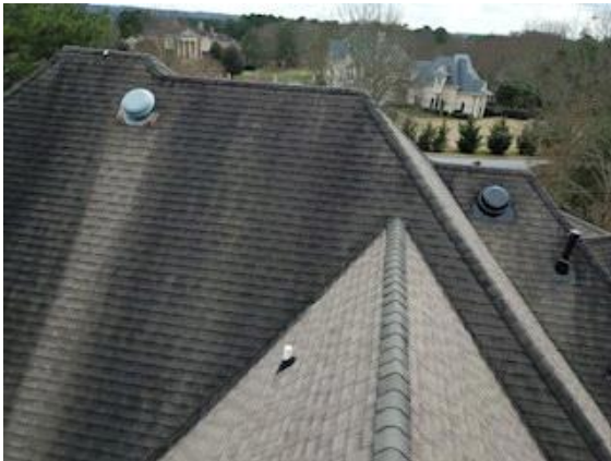
Roofing: Roof was exhibiting sign of aging, surface discoloration
