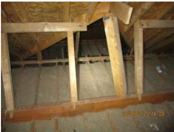
Attic Insulation: insufficient blown in insulation materials
