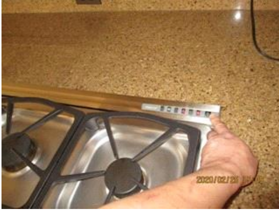
Kitchen @ main level : exhaust fan not operational
