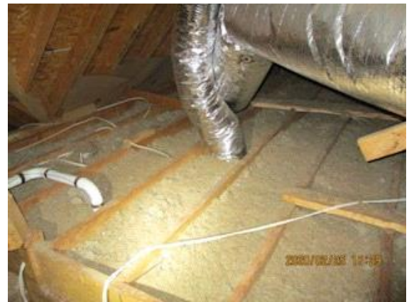
Attic Insulation: insufficient blown in insulation materials
