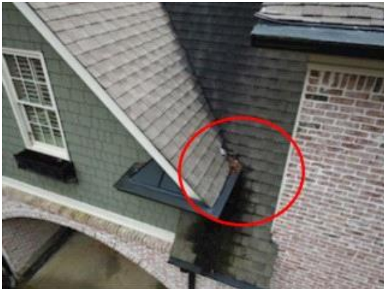
Gutters/Down Spouts: Gutter draining to the lower roof directly which could result in leakage
