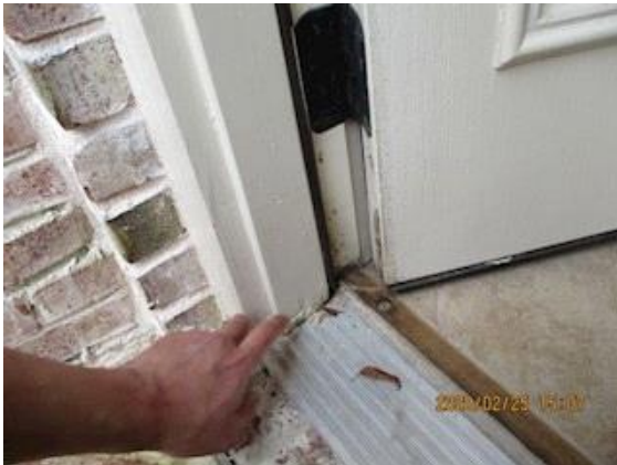
Exterior Doors: door jamb damaged near the bottom
