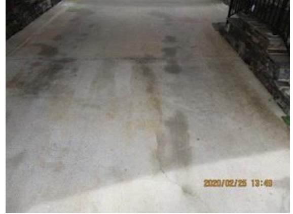
Driveway: cracked driveway surface
