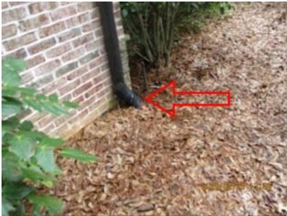
Gutters/Down Spouts: Downspout draining into subsurface, unable to locate the drainage outlet
