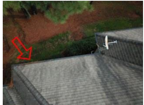
Gutters/Down Spouts: Gutter was full of debris
