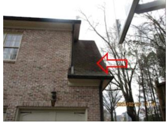
Roofing: moss / algae growth on the roof surface
