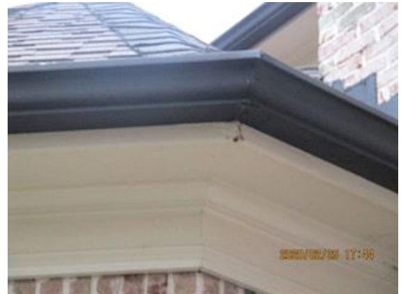
Gutter : gutter leaking water at the seam
