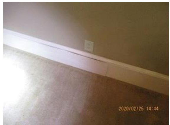
Basement grand room : water damages on the baseboard
