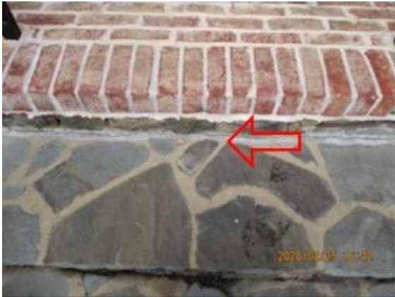
Walks / Steps: slight separation at the front stoop
