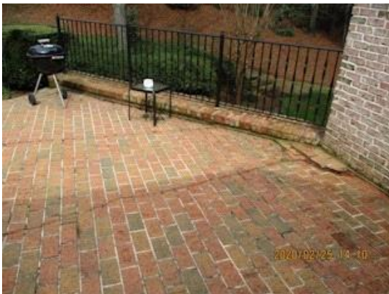
Patio: cracks and settlement
