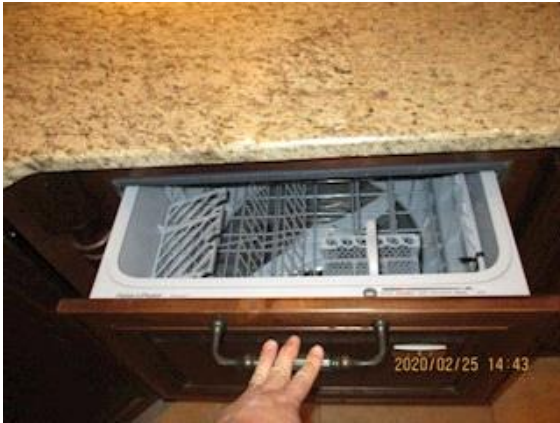
Kitchen @ basement : dishwasher not securely mounted into the cabinet
