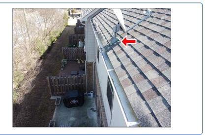
(2) Boot flashing around plumbing vents on the roof are ok now, but these last about 5-7 years before needing replacement. They crack and split and allow rain water to leak into attic. Check roof decking periodically for leaking into the inside the attic.
