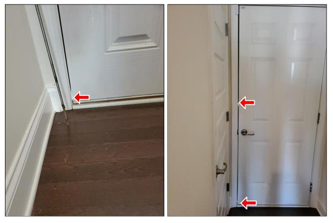
(2) Replace or re-attach torn weather strip at the underside of patio door.
