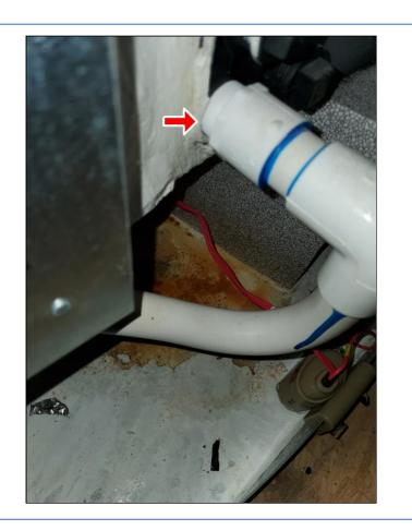
(2) Have the condensate drain line for the heat pump unit extend out and away from the home.
