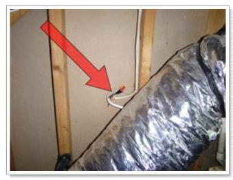
Uncovered electrical connections were noted in the attic behind the laundry and under the basement stairs. Recommend placing all electrical connections in covered junction boxes for safety.
