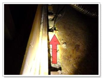
Uncovered electrical connections were noted in the attic behind the laundry and under the basement stairs. Recommend placing all electrical connections in covered junction boxes for safety.
