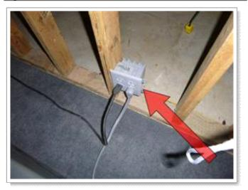
The basement bathroom outlet and the unfinished basement outlets are not GFCI protected. GFCI outlets are recommended on the exterior, in the garage, unfinished basement, crawlspace, and within 6 feet of sinks to prevent accidental electrical shock.
