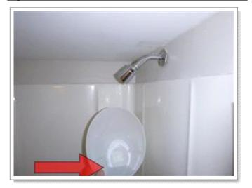
The basement shower head drips while the faucet is turned off. The waster supply plumbing for the shower is also leaking. Recommend inspection and repair by qualified plumber.
