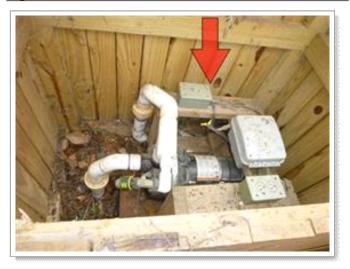
The sprinkler system was not operational. The electrical connector has been removed. There is an irrigation pump in the box on the lower patio which has no electrical connection. Recommend further evaluation and repair by qualified contractor.
