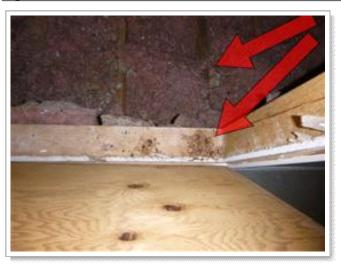
Evidence of animal infestation in the attic space above the garage hallway. Heavy wood roach evidence noted in the same space. Recommend consulting an exclusion/extermination service to seal all entry points and eliminate infestation.
