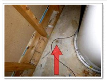
The basement shower head drips while the faucet is turned off. The waster supply plumbing for the shower is also leaking. Recommend inspection and repair by qualified plumber.
