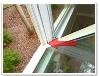
The lower rear window sash in the bonus room is not attached to the springs. This will keep the sash from staying up and allow the sash to fall suddenly. Recommend repair for security and safety.
