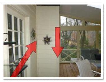
The screen porch is partially supported by the cantilevered chimney framing. The chimney has sagged. Recommend installing vertical posts supported by proper footings to prevent further sagging footings not present under walkway.
