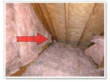
Evidence of animal infestation in the attic space above the garage hallway. Heavy wood roach evidence noted in the same space. Recommend consulting an exclusion/extermination service to seal all entry points and eliminate infestation.
