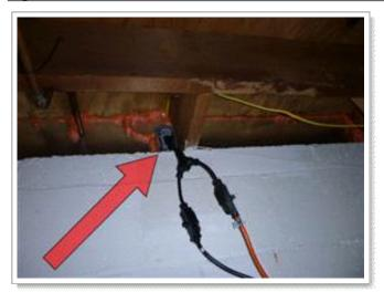
The basement bathroom outlet and the unfinished basement outlets are not GFCI protected. GFCI outlets are recommended on the exterior, in the garage, unfinished basement, crawlspace, and within 6 feet of sinks to prevent accidental electrical shock.
