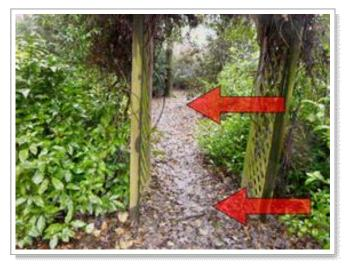
The walkway on the left side of the home also serves as drainage from the front yard. The area does not drain properly. Recommend proper grading/landscaping to allow for drainage.
