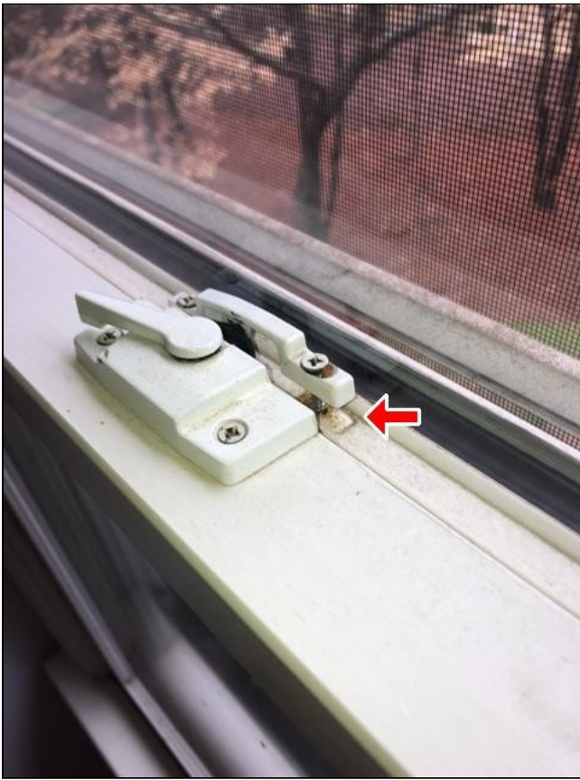
6.6 Second floor right rear corner bedroom
