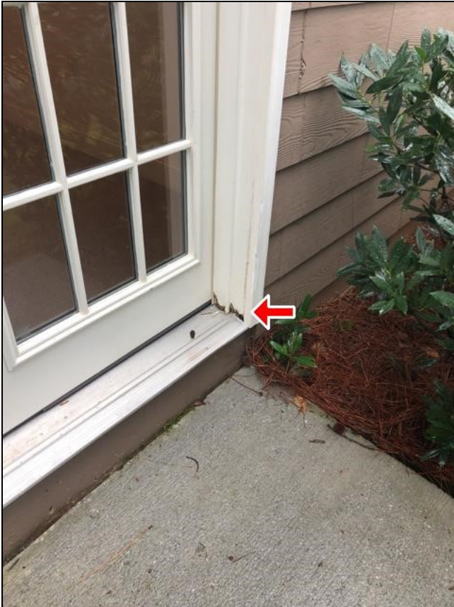
3.4 Basement door at rear of home
