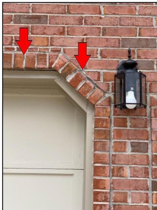
11. Mortar deterioration Task: Point repairs b...
