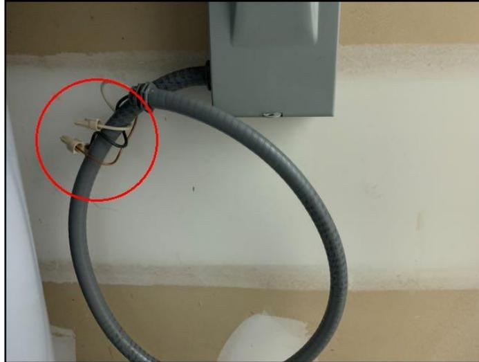
30. Abandoned Wiring Task: Remove Time:...
