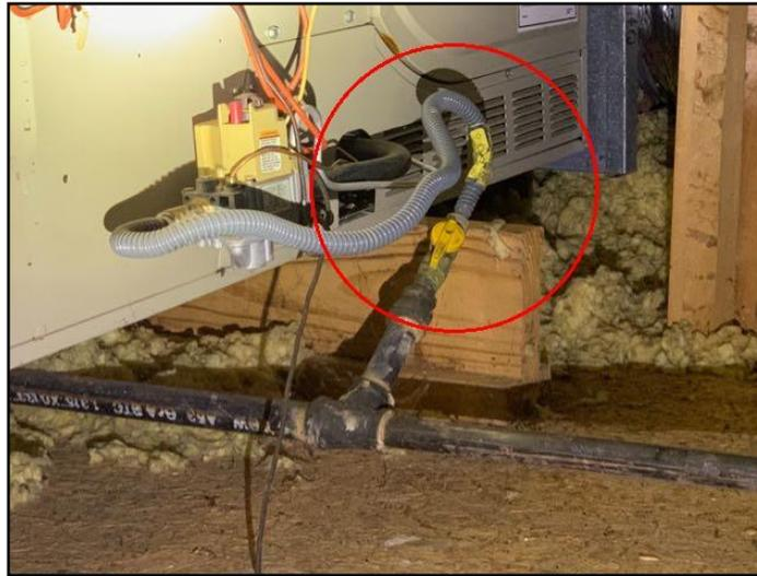
34. No drip leg (sediment trap, dirt pocket)
