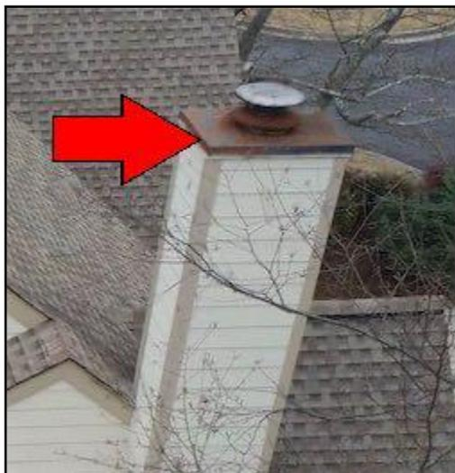
2. Chimney cap rusted or ponding Task: Repair...
