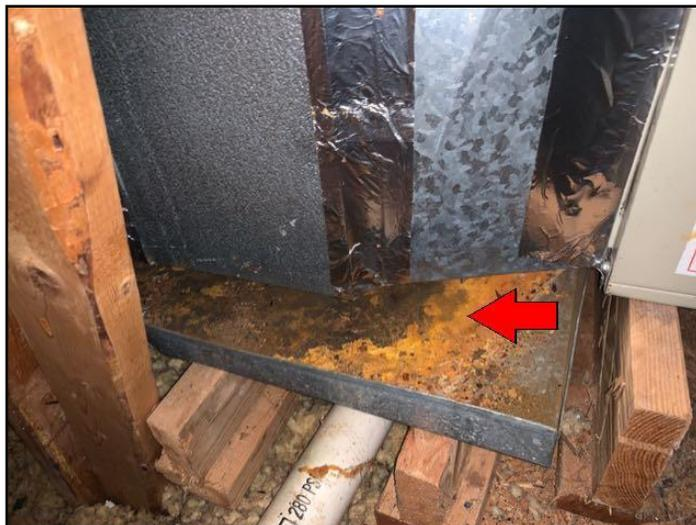
37. Auxiliary Pan Rusted Task: Replace Time:...
