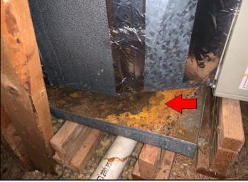
37. Auxiliary Pan Rusted Task: Replace Time:...
