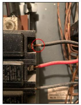
29. Not well secured Task: Secure Time:...
