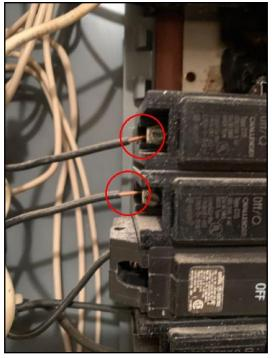
28. Not well secured Task: Secure Time:...
