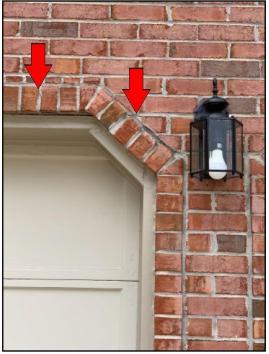
**11.** Mortar deterioration Task: Point repairs b...
