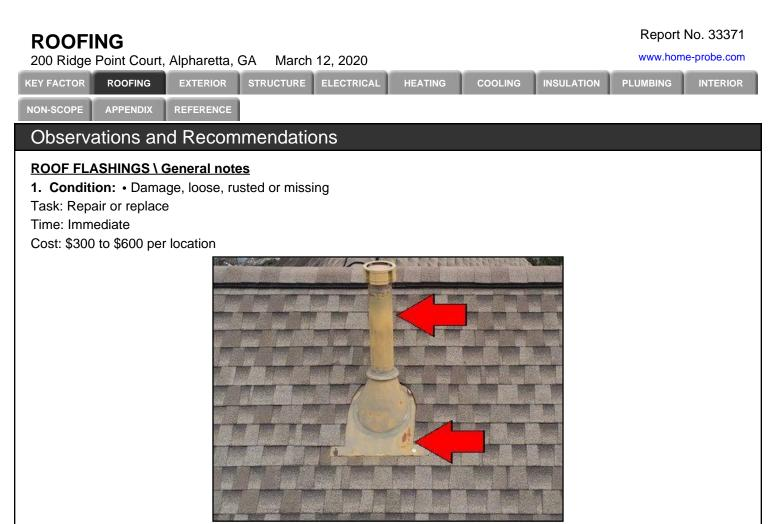
1. Damage, loose, rusted or missing Task:...
