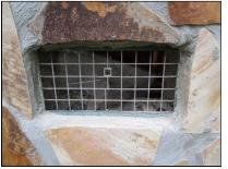
Replace damaged or missing small screens on the crawlspace vents.
