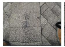
Repair cracked and damaged ridge cap shingles.
