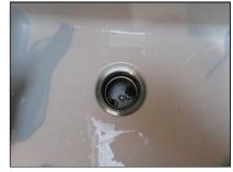
Replace the missing splash guard at the kitchen sink
