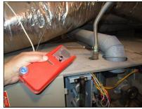
No gas leaks at the furnace.
