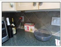
Add GFCI protection to the receptacle to the left of the sink
