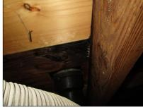
Stained decking below the flue and above the plumbing vent
