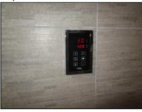
Display indicated an EO error and the unit shut down
