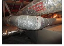
Rust on the flue in the crawlspace, replace damaged flue.
