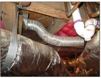
Replace flex dryer vent with solid pipe.
