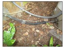
Replace the damaged insulation on the condensing unit.
