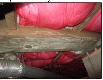
Common fungal growth on the joists in the crawlspace.
