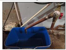
Extend the T/P drain line to the exterior of the house.
