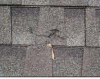
Repair damaged shingles, damaged by tree branches.
