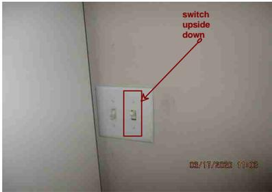
The two three way switches which operate the ceiling light in the laundry room are not properly wired. A licensed electrician should evaluate for repair.
