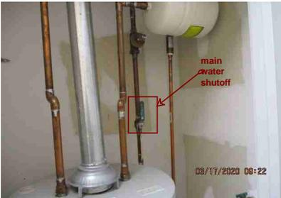
The water pressure tested 100 psi at 9:25 a.m..
