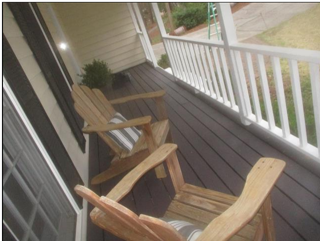
1.3 Item 1(Picture) Front porch has settled and leans downward
