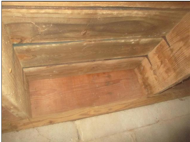
1.3 Item 4(Picture) Front porch is nailed to home, modern deck type installations would be bolted to home
