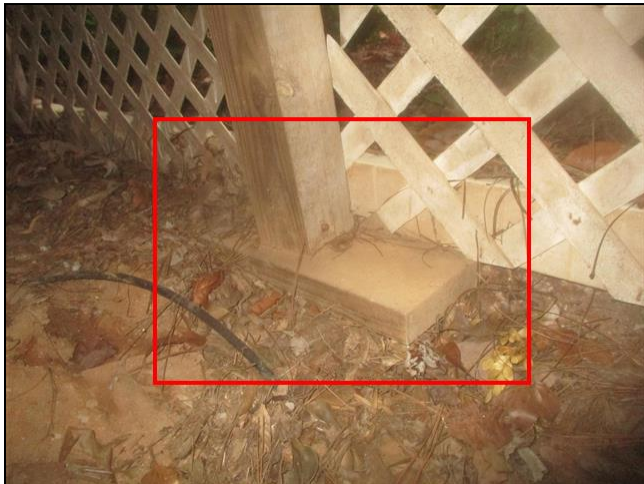
1.3 Item 3(Picture) Most front columns are on loose/ above ground wood footings (modern deck columns would have buried concrete footings)
