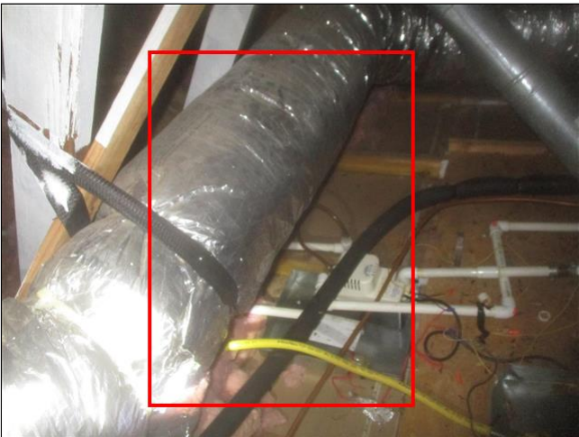
5.0 Item 2(Picture) Missing insulation, central attic location
