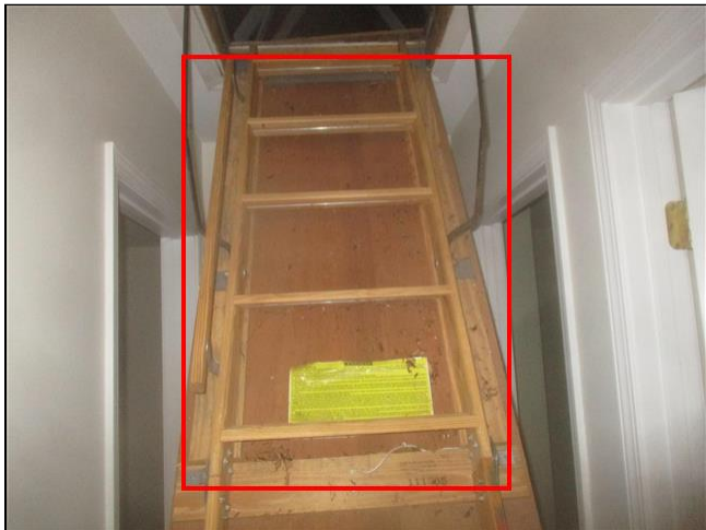
5.0 Item 1(Picture) Insulate attic pull down stairs
