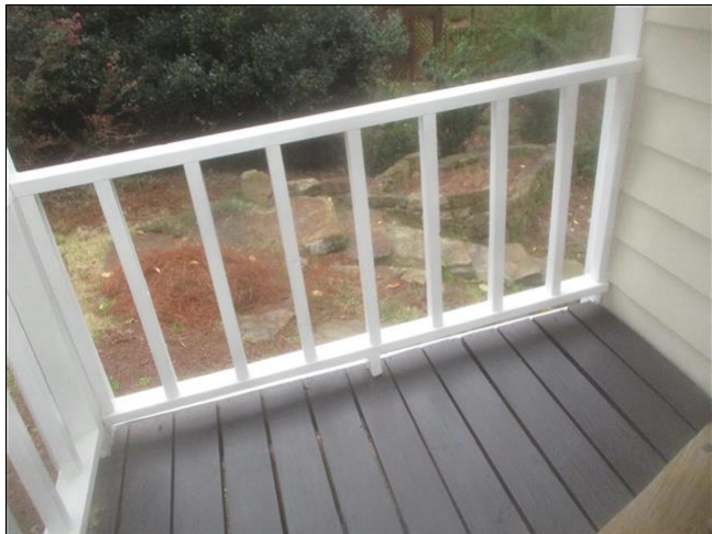
1.3 Item 2(Picture) Spindles for front porch are greater than 4 inches apart (safety concern for small children)
