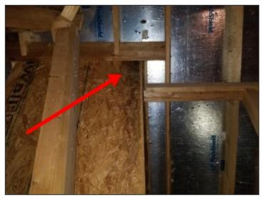
Evidence of a leak at front chimney corner
