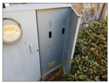
Main electrical disconnects at exterior meter
