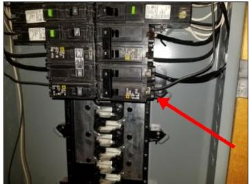
Improper wire size at bottom right 35 amp breaker in panel A
