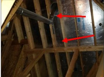
Evidence of a leak at second floor furnace exhaust vent penetration
