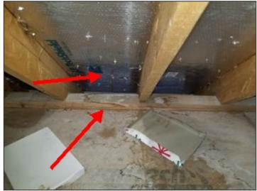
Evidence of a previous leak at left small master closet attic space
