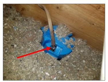
Burned electrical wire in attic above loft bathroom
