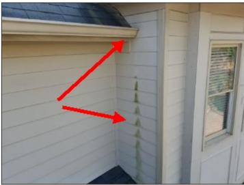
Improper gutter slope at garage roof
