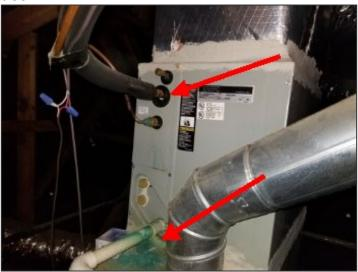
Coolant line not fully insulated at evaporator
