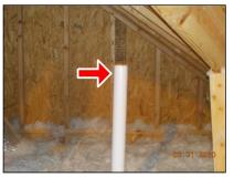
Plumbing vent piping terminates in the attic
