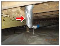
The dryer exhaust vent uses flexible metal piping running through the crawlspace.
