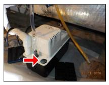
Cleaning the condensate pump reservoir and flushing the line with water is recommended at least twice a year
