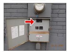
The main electrical disconnect is located at the meter.
