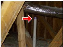
Plumbing vent piping terminates in the attic
