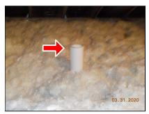
Plumbing vent piping terminates in the attic
