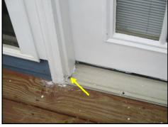
Moisture damage observed at the french doors on the left side of the house
