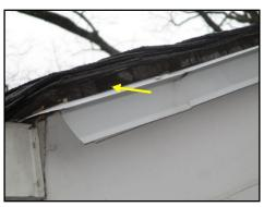
Wood rot observed on the roof decking on the front of the house
