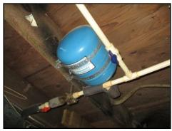
Expansion tank observed near the pressure regulator
