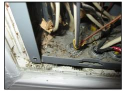
Rodent droppings observed inside of the gas furnace
