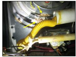
Rust observed inside of the gas furnace
