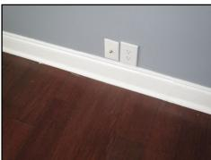
The outlets in the back right bedroom was installed less than 6" off the ground
