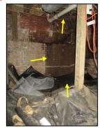
The Whirlpool dishwasher appeared to be Water leak observed in the crawlspace below the dishwasher
