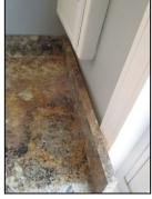
Gap observed around the back spash in the rear bathroom
