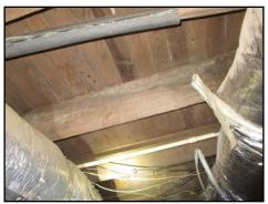
Suspected Microbial growth observed on the structural members in the crawlspace
