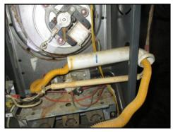
Flexible gas line observed inside of the gas furnace
