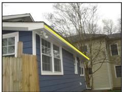
Missing gutters observed on the back of the house
