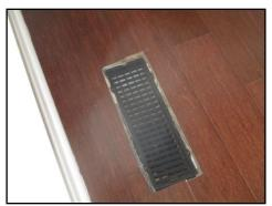
Improper fitting register observed in the middle bedroom on the right side of the house
