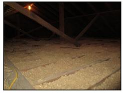
Thin insulation observed in the attic space
