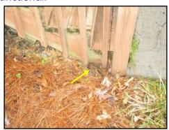
Wood to ground contact observed on the wood steps on the front of the house
