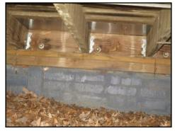
Proper flashing observed below the front porch decking
