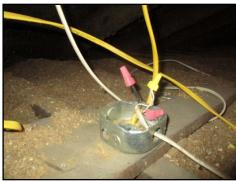
Wire connection observed outside of a junction box
