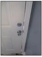
Daylight observed around the rear door when the dead bolt was not locked
