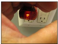
The outlets in the master bathroom did not appear to be wired properly
