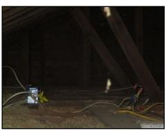
Wire connections made outside of the junction boxes
