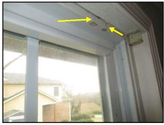
Water staining observed in the rear bathroom window
