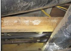
Suspected Microbial growth observed on the structural members in the crawlspace
