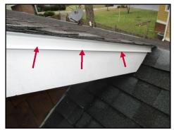
Areas of missing drip edge flashing on the back of Drip edge flashing observed on the front of the house
