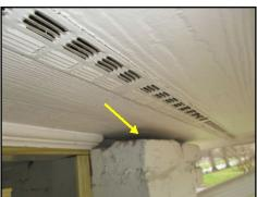
Open construction gap observed on the front porch
