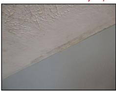
Suspected Microbial growth observed on the ceiling in the rear bathroom
