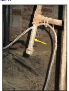
Sediment trap observed at the gas furnace
