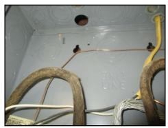
Missing grommet observed in the top of the electrical panel
