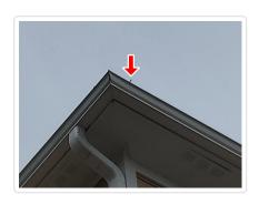
• Repair Requested Seller to have roofer re-nail the gutters to the fascia.
