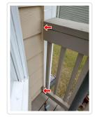
Repair Requested Securely attach deck guard rail to house.
