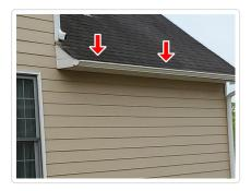
• Repair Requested Seller to have roofer repair and re-nail gutter to the fascia after roof is replaced.
