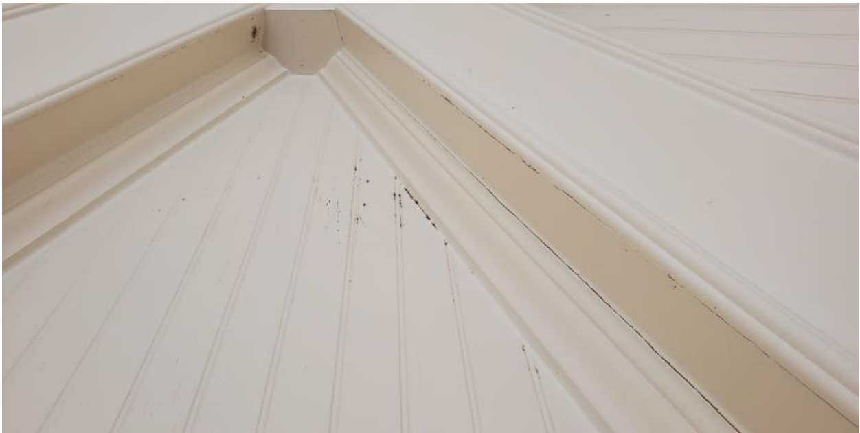
3. Kitchen Dining room crack and mold
