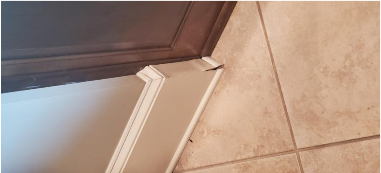
4. Basement Bar base board rod water damage
