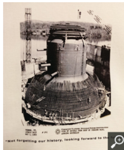
A view of Vermont Yankee Nuclear Power Plant in 1969 shows construction of the drywell.
