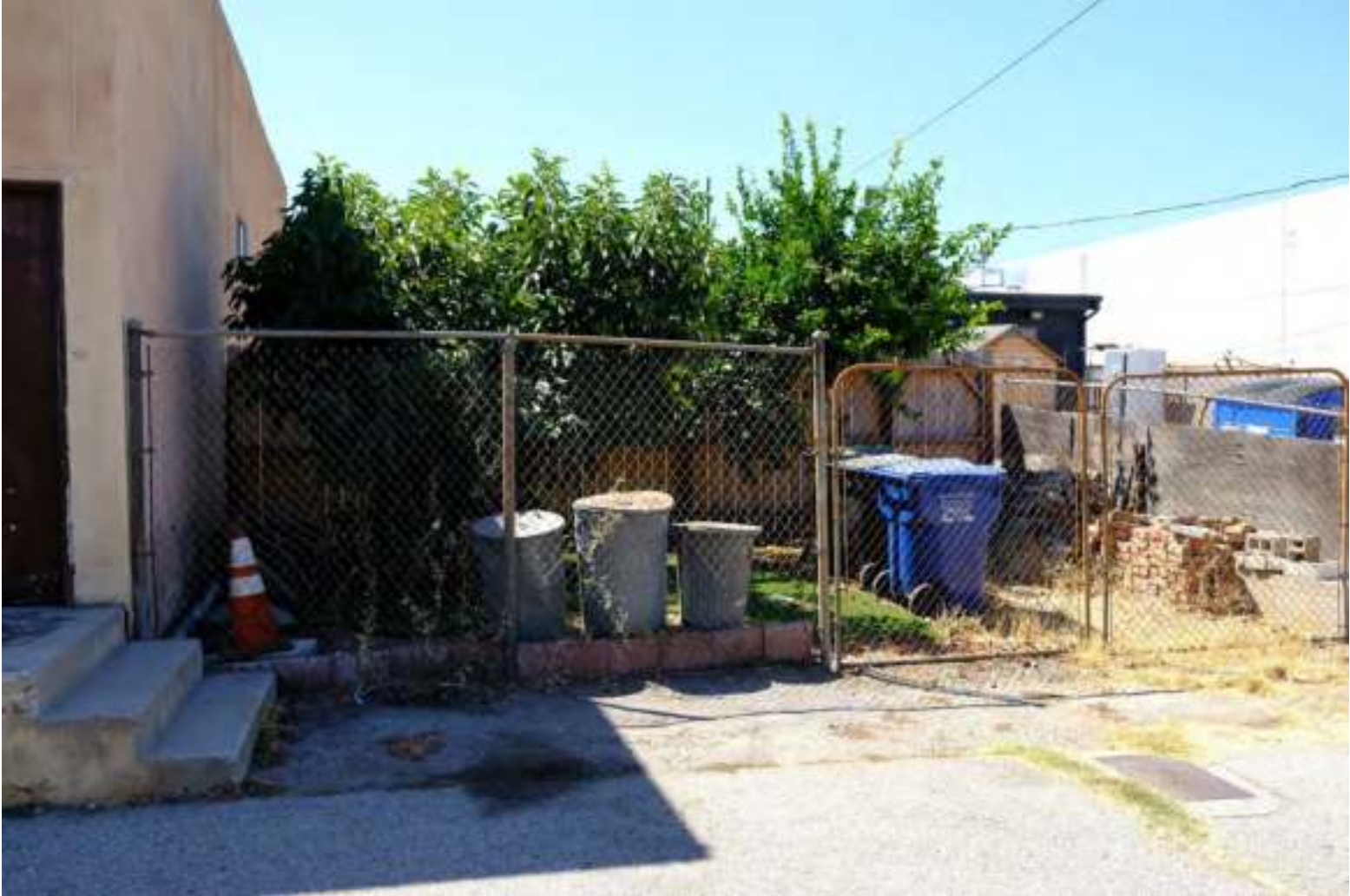
Jay Risk Standard Oil Co. Service Station. View south from the alley. (Luftman 2022)
