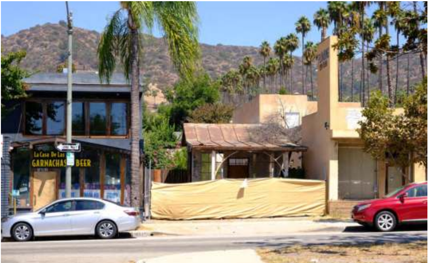
Jay Risk Standard Oil Co. Service Station. View north. Photographed after the owner started to disassemble the building. (Luftman 2022)
